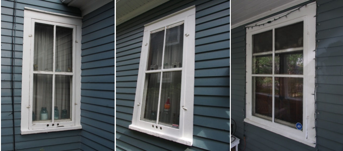
(Image #2.8 – Remaining one-over-one sash windows with storm sashes)
