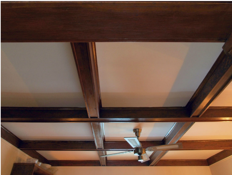
(Image #3.3 – Detail of decorative ceiling beams)
