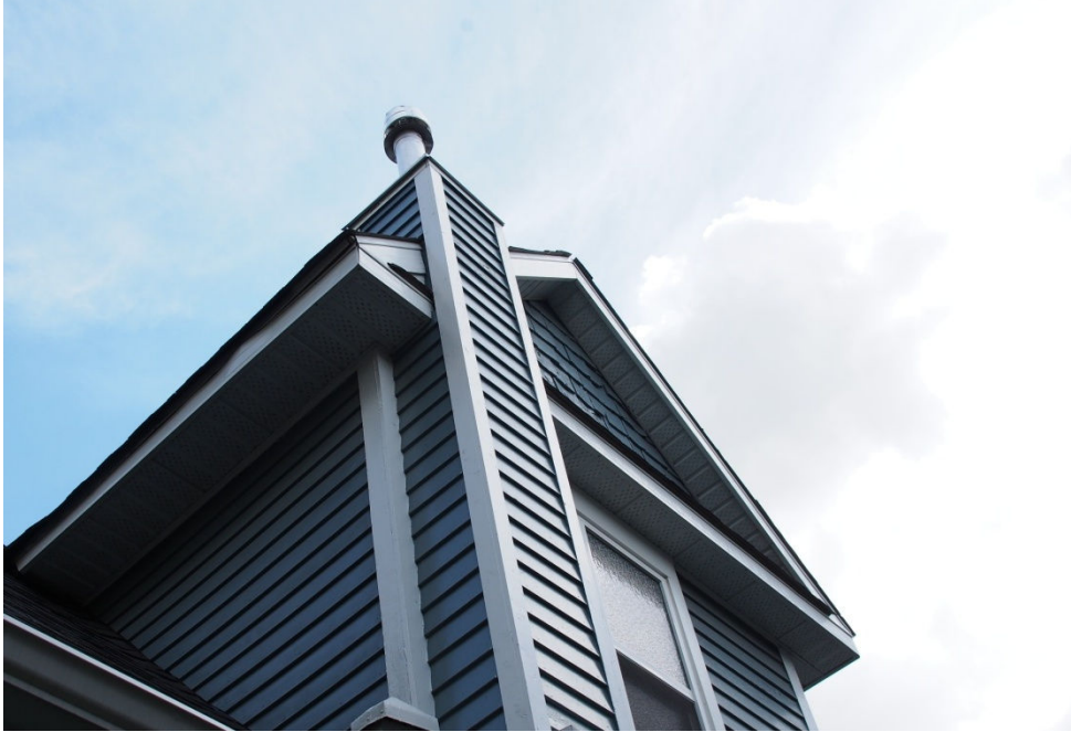
(Image #2.6 – West façade dormer, showing wood shingles on gable-front)
