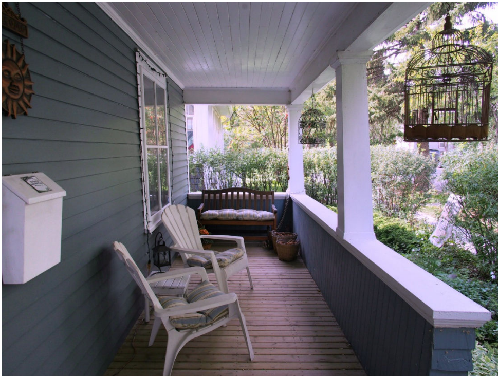
(Image #2.7 – Front porch, showing support posts, balustrade, tongue-and-groove ceiling)
