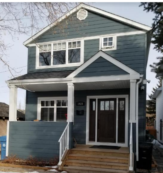
1428 1A ST NW, renovated c.1913 2-story home, immediately adjacent to proposal for 6-storeys
