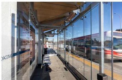
Photo: Transit stops and infrastructure should be integrated with the sidewalk safely and conveniently.
