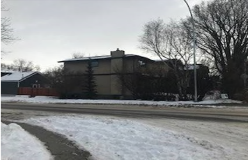
This is the house directly across 5 th Street from 602
