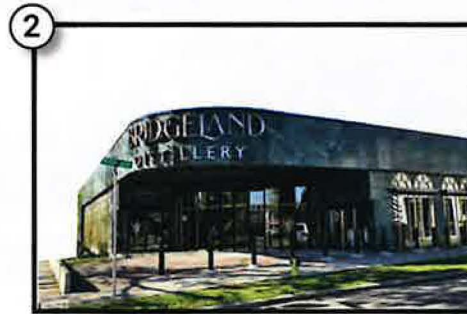
2 Bridgeland Distillery Refurbished Commercial
