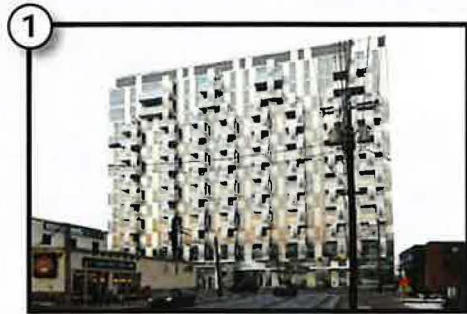
1 Era by Minto Under Construction
