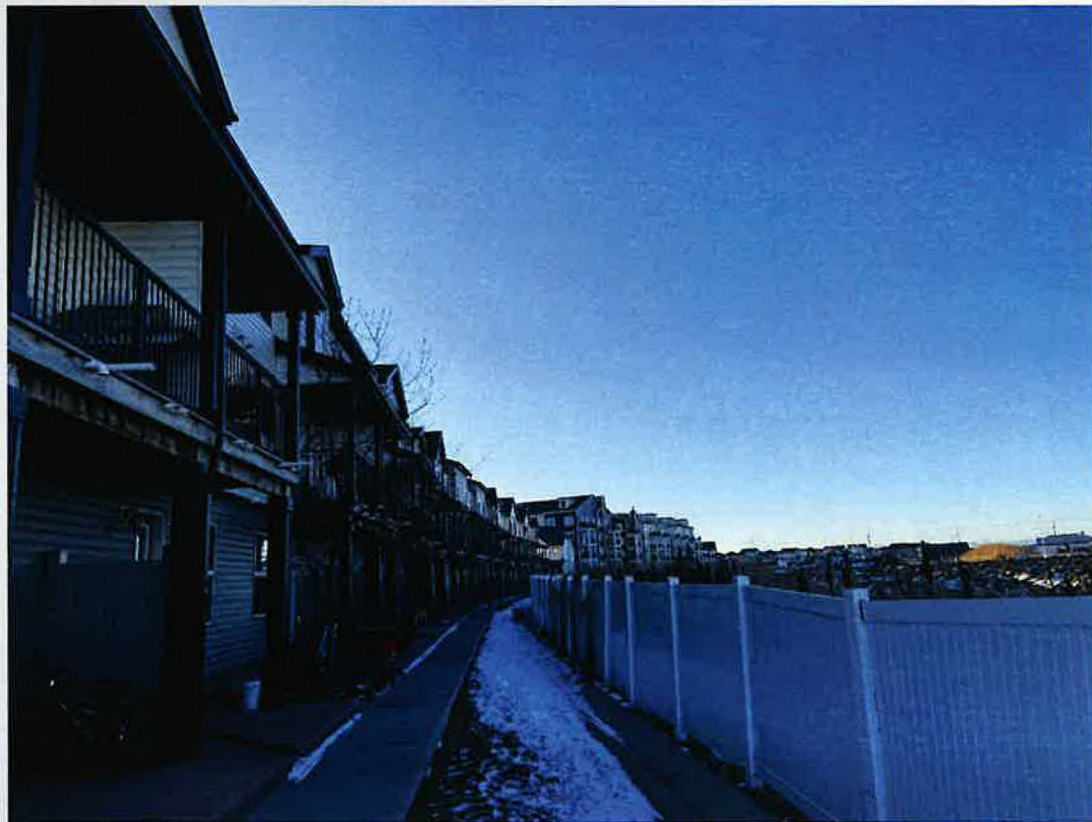
North side (facing site)
