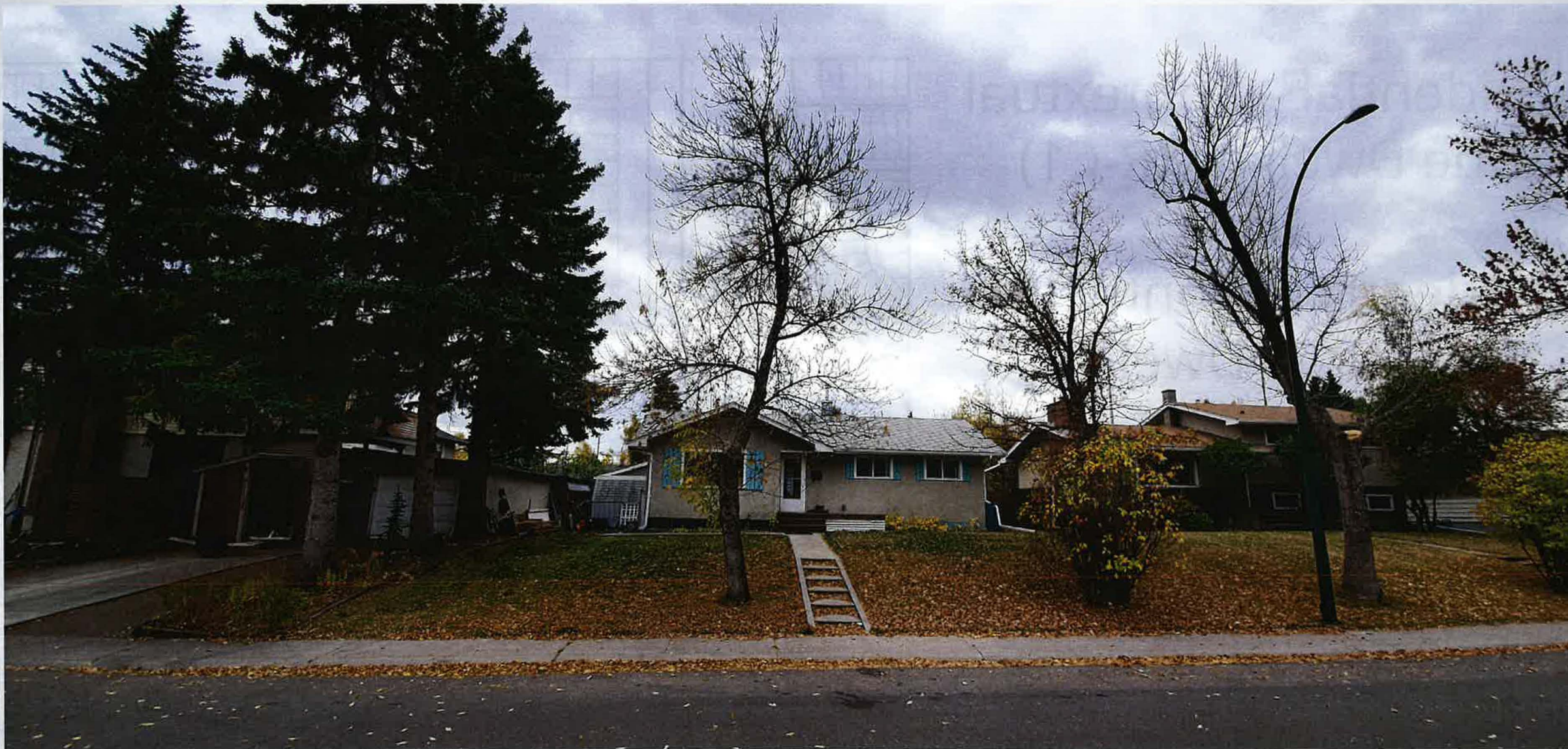
View of the front, looking southwest.
