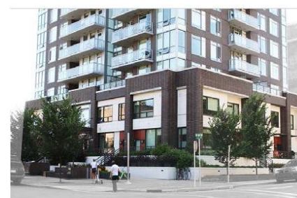
Photo: A building with a clearly defined base and distinct upper portions that reinforce the street wall .
