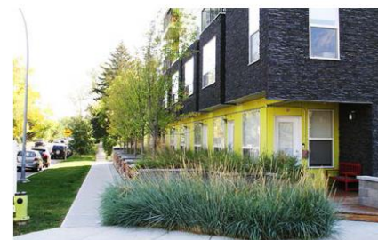
Photo: This residential frontage provides well-marked entrances for each unit, and wraps the materials and landscape features around the building corner.
