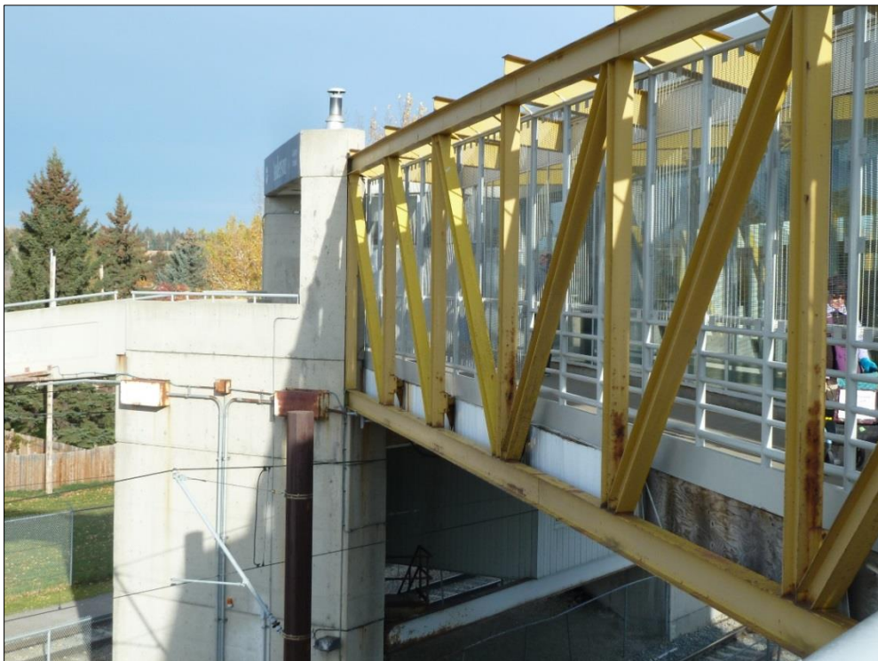
Figure 13: Paint peeling off on steel truss
