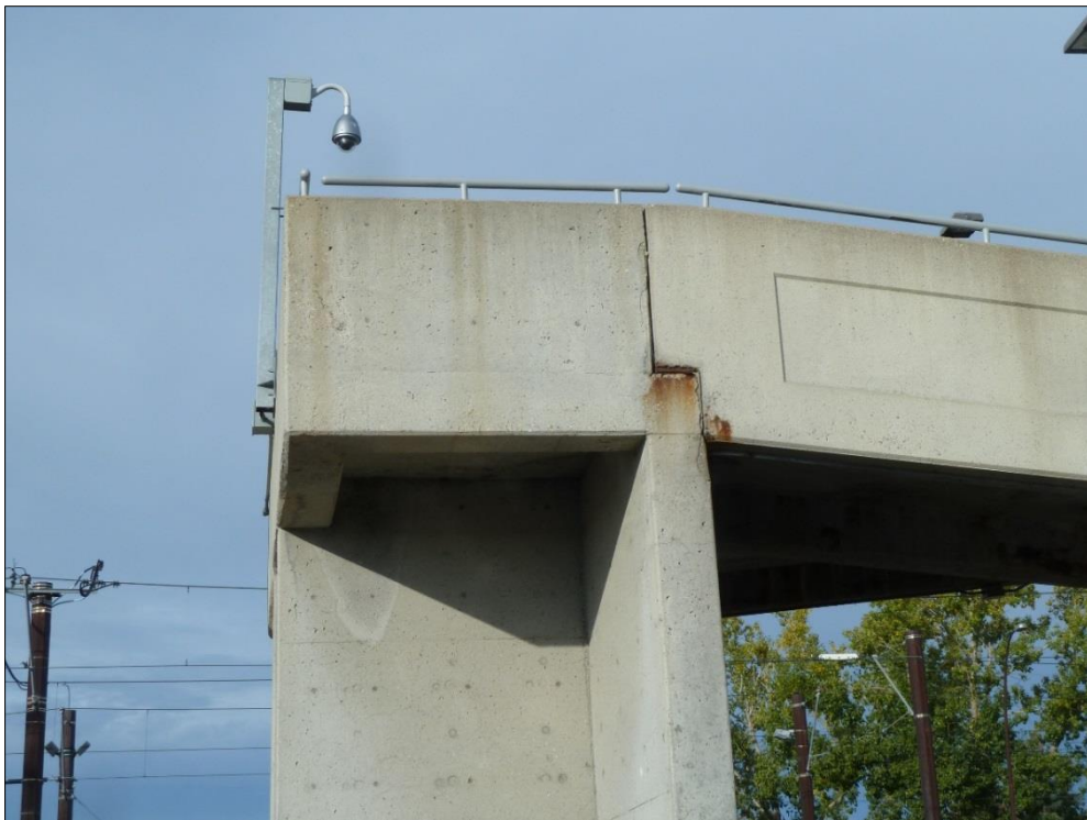
Figure 10: East Ramp Pier - Rust stains
