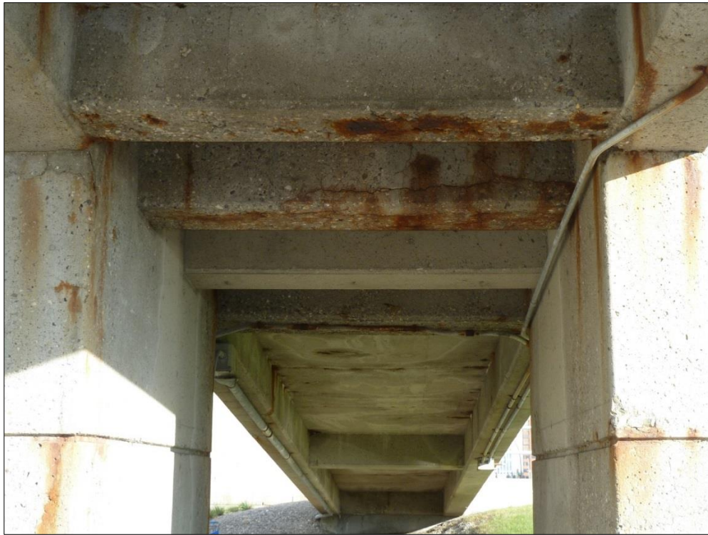
Figure 7: East Ramp Soffit - Longitudinal cracks, rust stains
