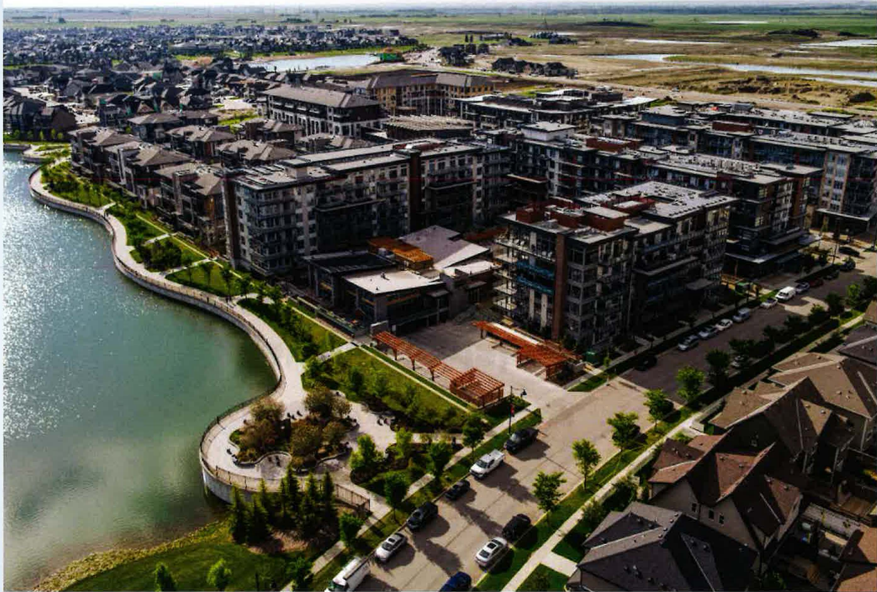
Westman Village – Aerial looking southeast
