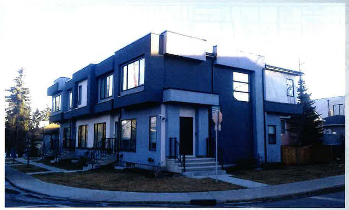
Existing rowhouse along 32 Avenue NE (R-CG District)
