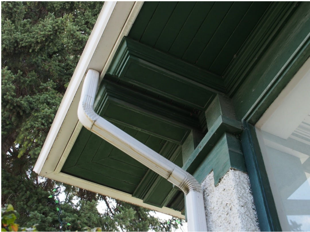
(Image #2.9 – Example of column capital with eave brackets)
