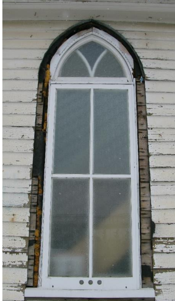
(Images 2.8 and 2.9: Examples of typical 2-over-2 double-hung wooden-sash window with 3-light fixed stained glass, gothic-arched transoms and wooden lug sills; 4-light wooden storm window. Note: finishing wooden trim uninstalled)
