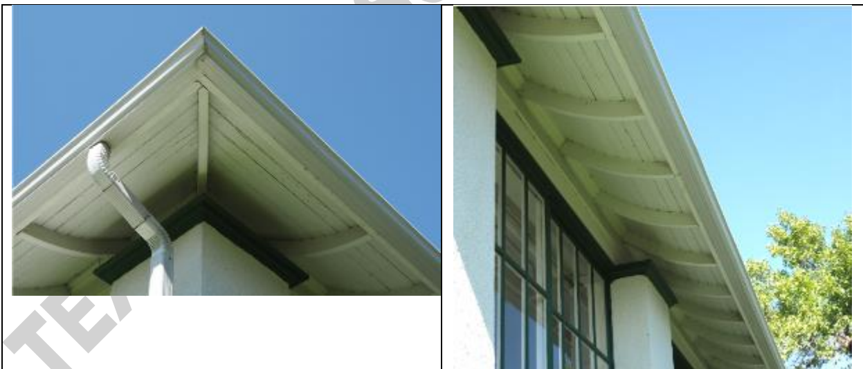
Images 2.8 and 2.9: Examples of projecting eaves with exposed curved rafter tails and wood tongue-and-groove soffits; plain wood fascia
