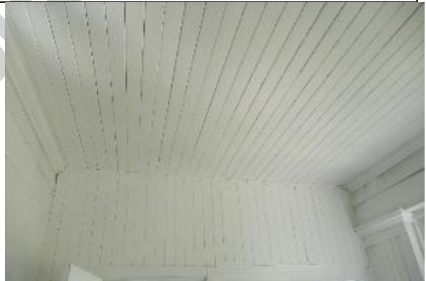
Image 3.5: Example of the tongue and groove wood ceiling and dividing wall
