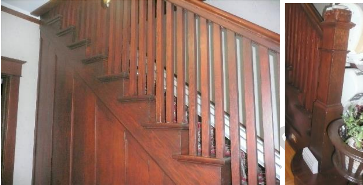
(Images 3.10 and 3.11: Wood paneled stair wall and balustrade with square newel post on rounded riser)
