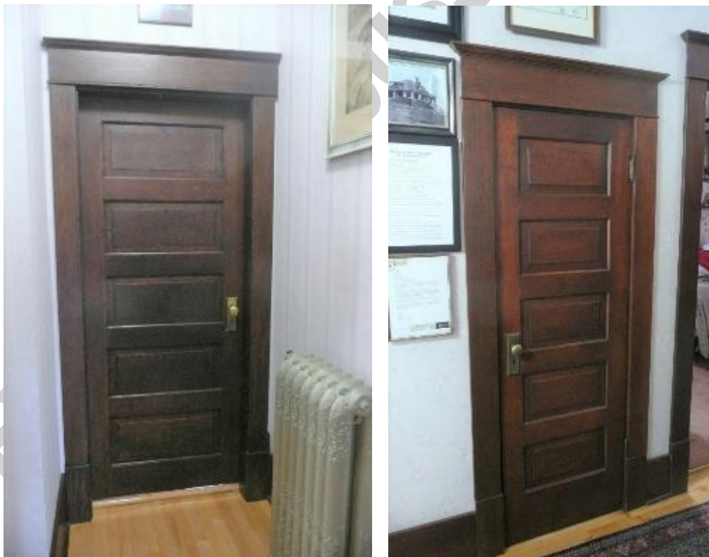
(Images 3.12 and 3.13: Examples of wood trim, baseboards and extant interior 5-panel door)
