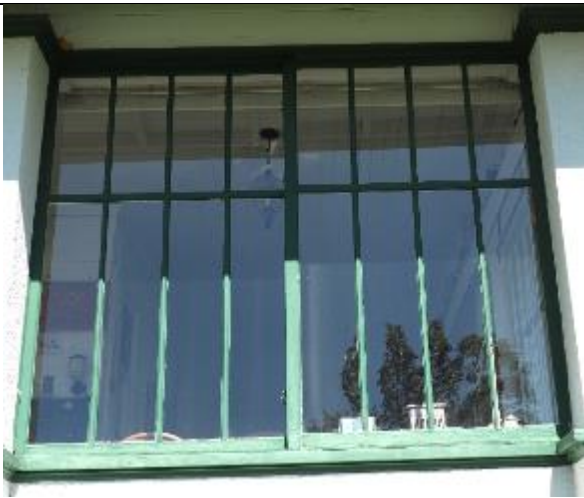
Image 2.15: Example of a 4-over-4 light wood slider windows of enclosed porch
