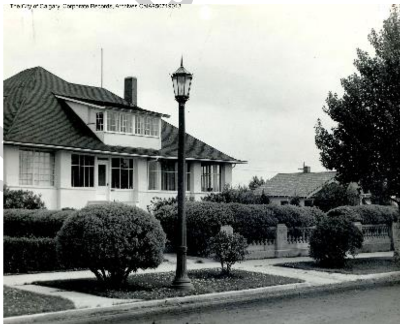
(Image 2.2: Historic image ca.1929. View of south façade showing porch and shed dormer balcony enclosed, and roughcast stucco cladding applied)
