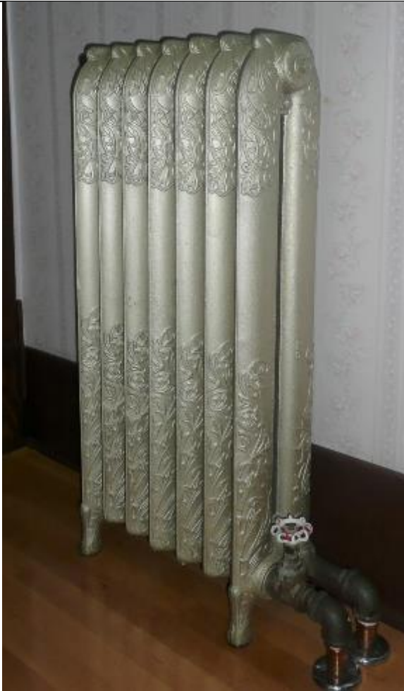
Image 3.17: Example of an in-situ cast iron radiator
