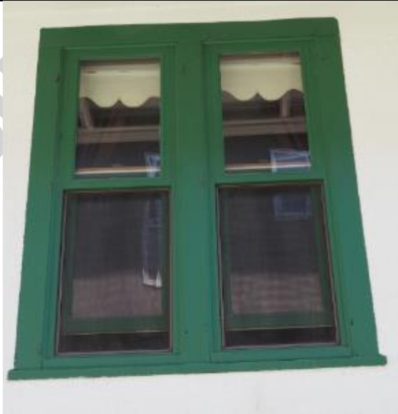
Image 2.16: Example of a 5-over-5 light wood windows of enclosed porch
