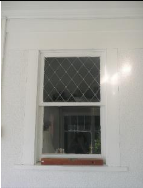
Image 3.2: Example of a 1-over-1 wood window with diamond shaped divided light upper sash
