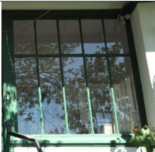
Image 2.16: Example of a 5-over-5 light wood windows of enclosed porch
