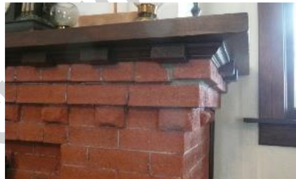
Images 3.18 and 3.19: Example of one of two identical brick fireplaces with wood mantels and decorative corbelling
