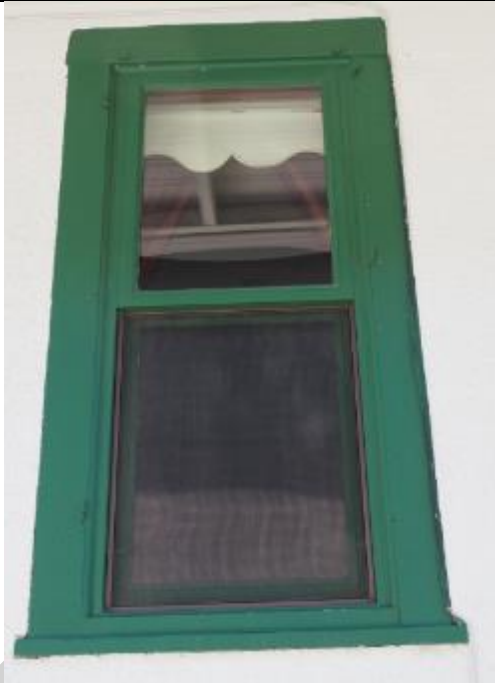
Image 2.17: Example of a 1-over-1 single assembly windows (west and north facades)
