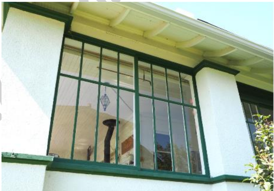
Image 2.14: Example of squared support columns from ground level terminating under the eaves with molded wood trim at caps; continuous molded wood band at balustrade level
