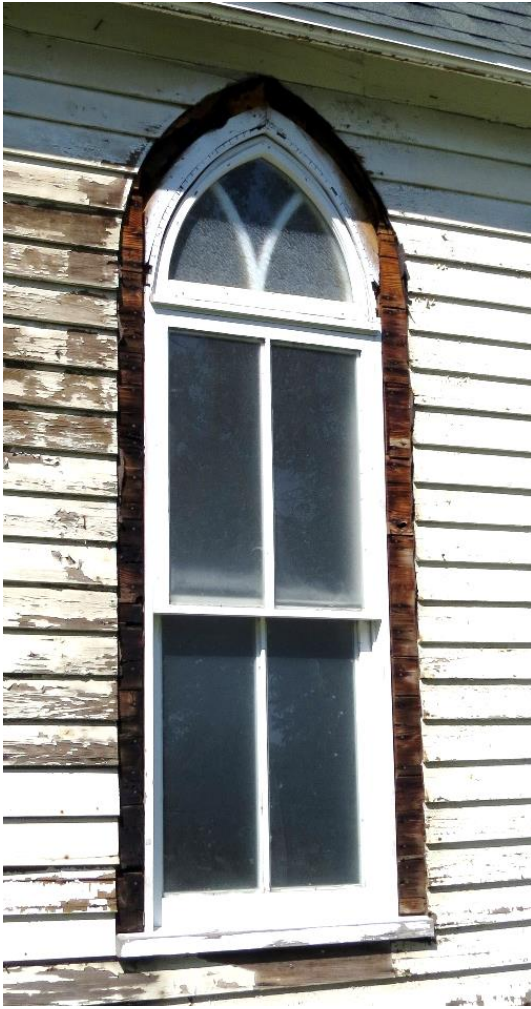
(Images 2.8 and 2.9: Examples of typical 2-over-2 double-hung wooden-sash window with 3-light fixed stained glass, gothic-arched transoms and wooden lug sills; 4-light wooden storm window. Note: finishing wooden trim uninstalled)
