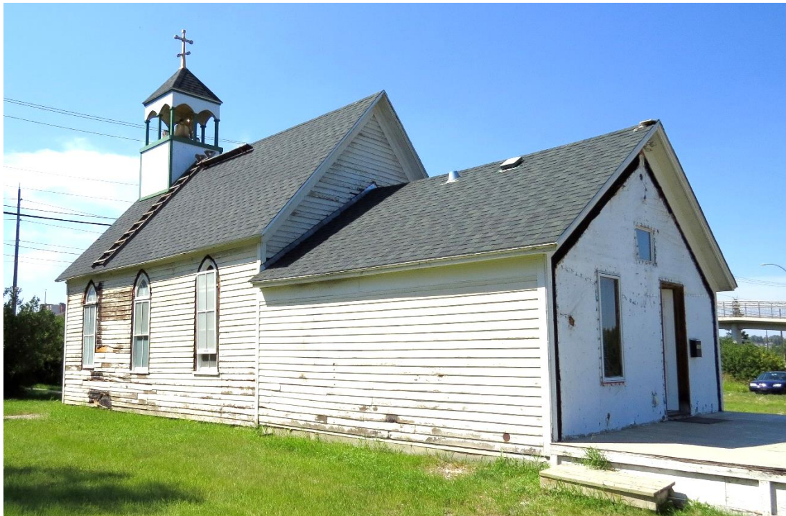
(Image 2.5: Oblique view showing east and south façade)
