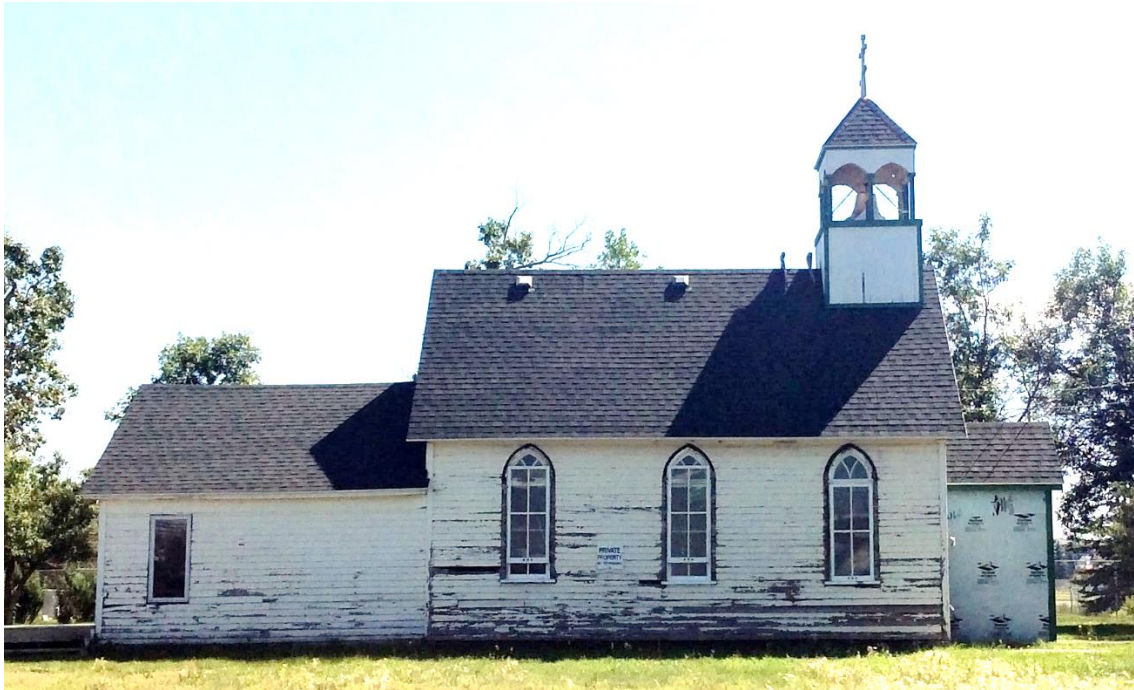
(Image 2.4: North façade)
