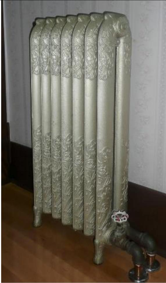
Image 3.17: Example of an in-situ cast iron radiator
