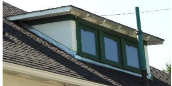
2.13: North dormer with flat roof and exposed wood rafter tails with decorative ends; triple assembly wood frame windows
