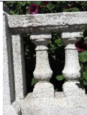
Images 1.3-1.5: details of the ornamental design with balustrade consisting of evenly spaced cast balusters with nine rectangular baluster posts
