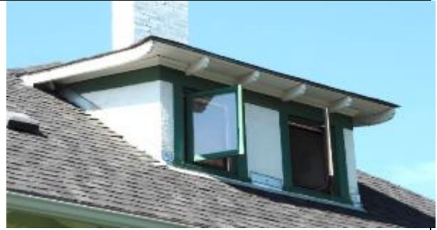
Image 2.11: Example of east and west shed dormer with flared roof and exposed wood curved rafter tails with decorative ends; triple assembly wood frame windows
