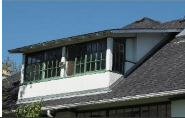
Image 2.10: South dormer with flat roof and exposed wood rafter tails with decorative ends; 12-light slider wood windows
