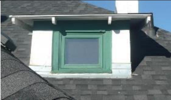
Image 2.12: Small East dormer with flat roof and exposed wood rafter tails with decorative ends; one wood frame window
