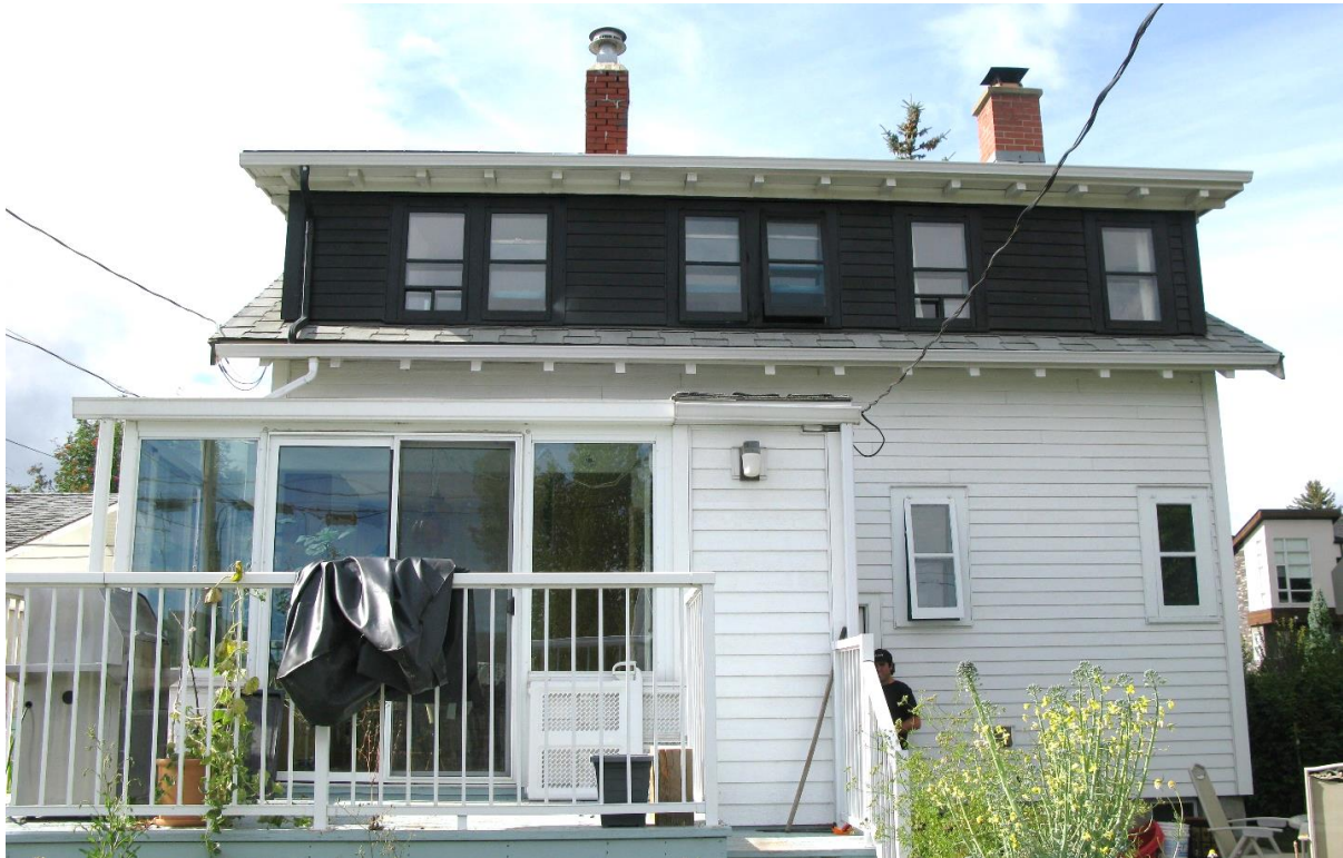
(Image 2.7: Southeast façade showing shed roof extension with six original 1-over-1 wood windows, four of which are in double assemblies. Note: Main floor façade on southeast façade is not regulated below the gabled roof line eaves)
