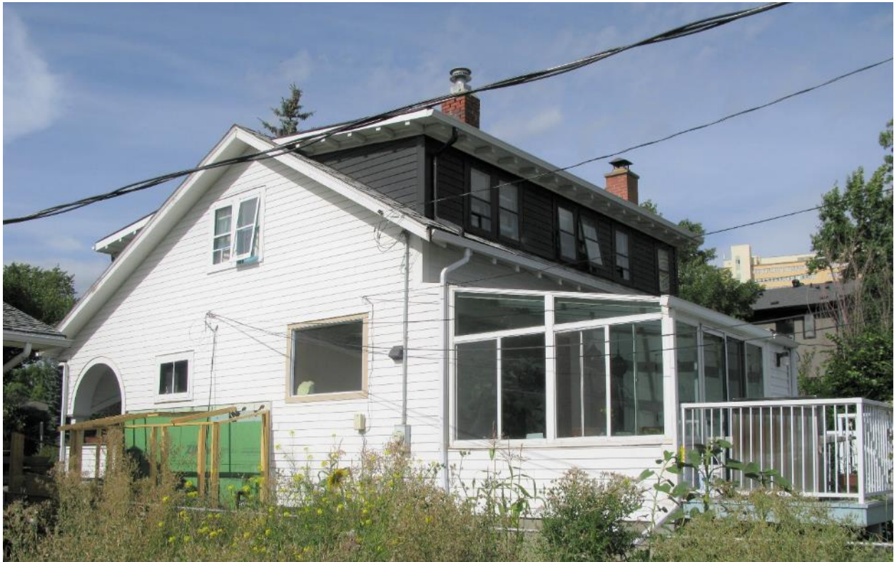
(Image 2.8: Southwest façade showing a double assembly of 1-over-1 wood windows; single fixed window; curved opening on side of porch)
