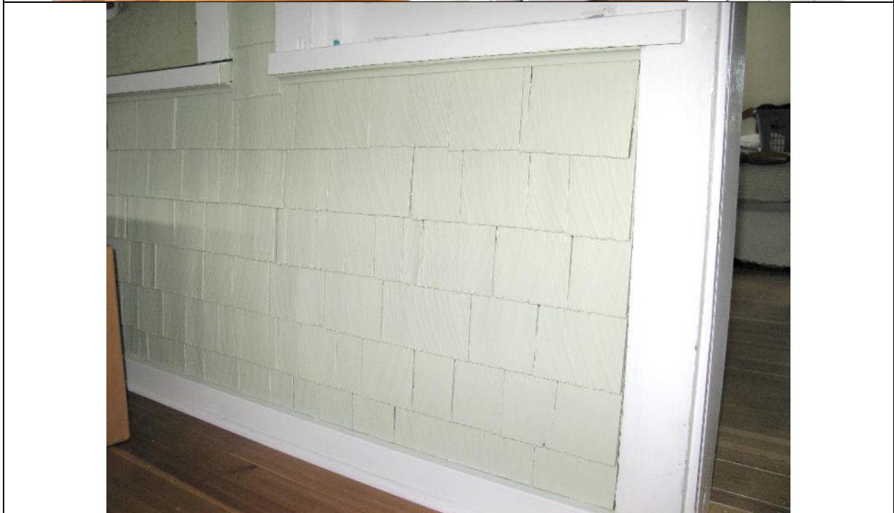
Images 3.9 and 3.10: Original balcony area consisted of mirrored fenestraion with four wood 1-over-1 single hung windows and two panelled doors with 2-over-2 lights; detail of original wood shingle cladding
