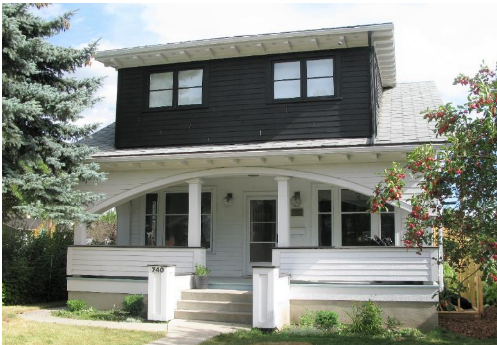
(Image 2.5: Northwest façade showing six original wood windows composed into two triple assemblies on the main floor; sweeping curved opening on porch)
