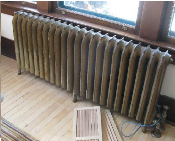
(Image 3.8: Example of cast iron radiator)
