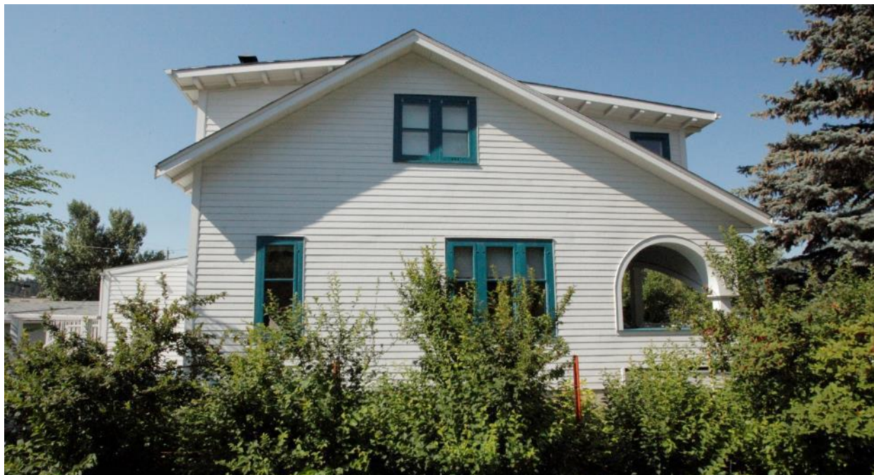
(Image 2.6: Northeast façade showing six 1-over-1 wood windows, three of which are in a triple assembly and two in a double assembly; curved opening on side of porch)
