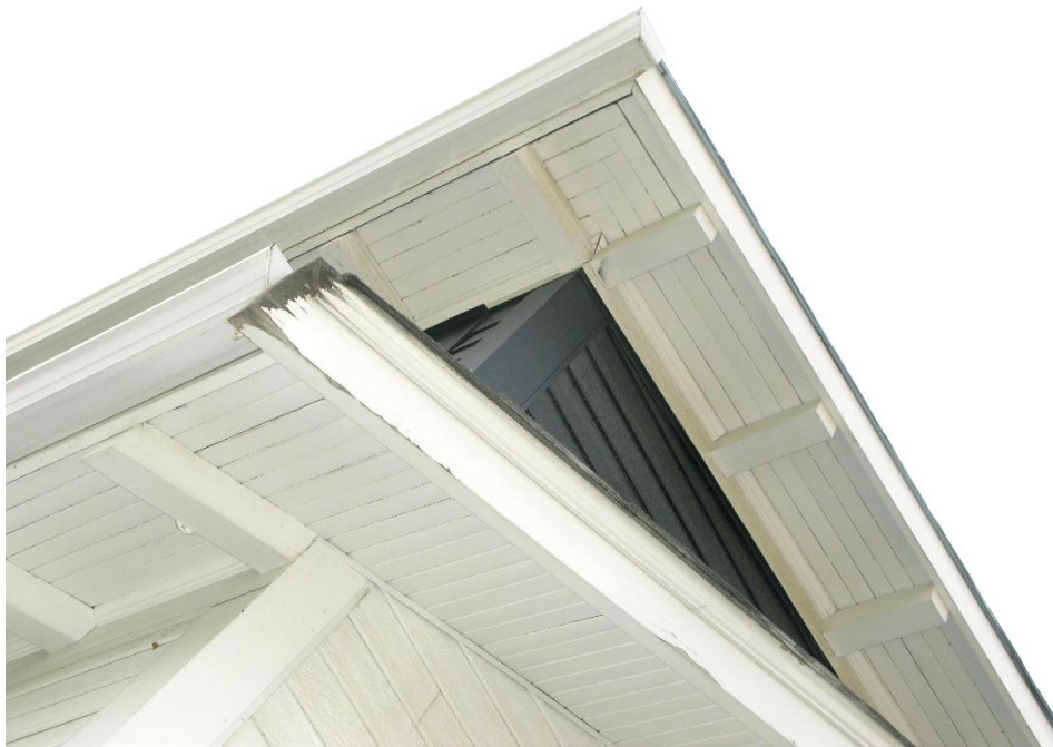
(Image 2.9: detail of typical wood eaves with exposed wood rafter tails with squared (shed roof extensions) or beveled ends (gabled roof); plain wood fascia; wood tongue-and-groove soffits)
