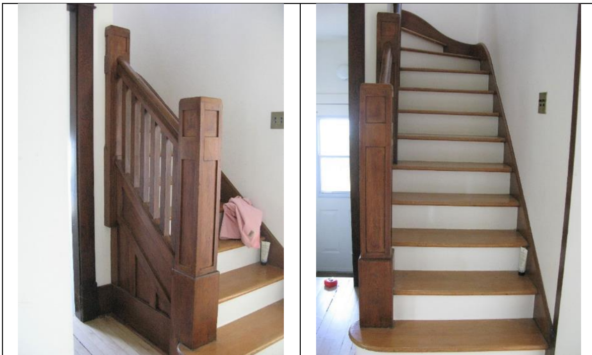
(Images 3.1 and 3.2: staircase with wood balustrade; paneled square newel posts and wall)
