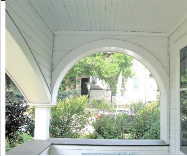
Image 2.10: Example showing curved opening on sides of front porch
