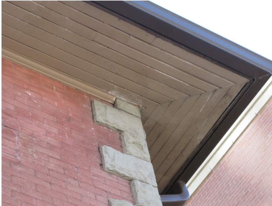
Photo 6.1: an example of the wooden tongue-and-groove soffits and cornices
