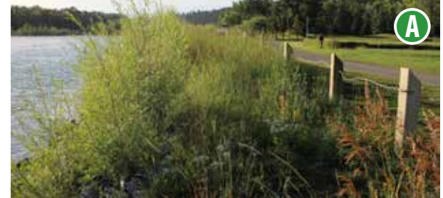
Vegetated rip rap – outfall B134
