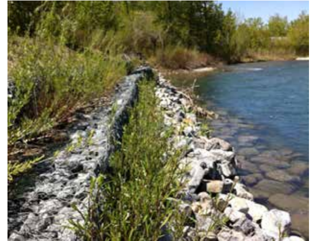
Vegetated gabion project
