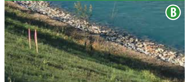
Home Road bank stabilization
