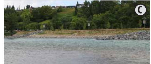
Rip rap and groynes – Sunnyside, Memorial Drive
