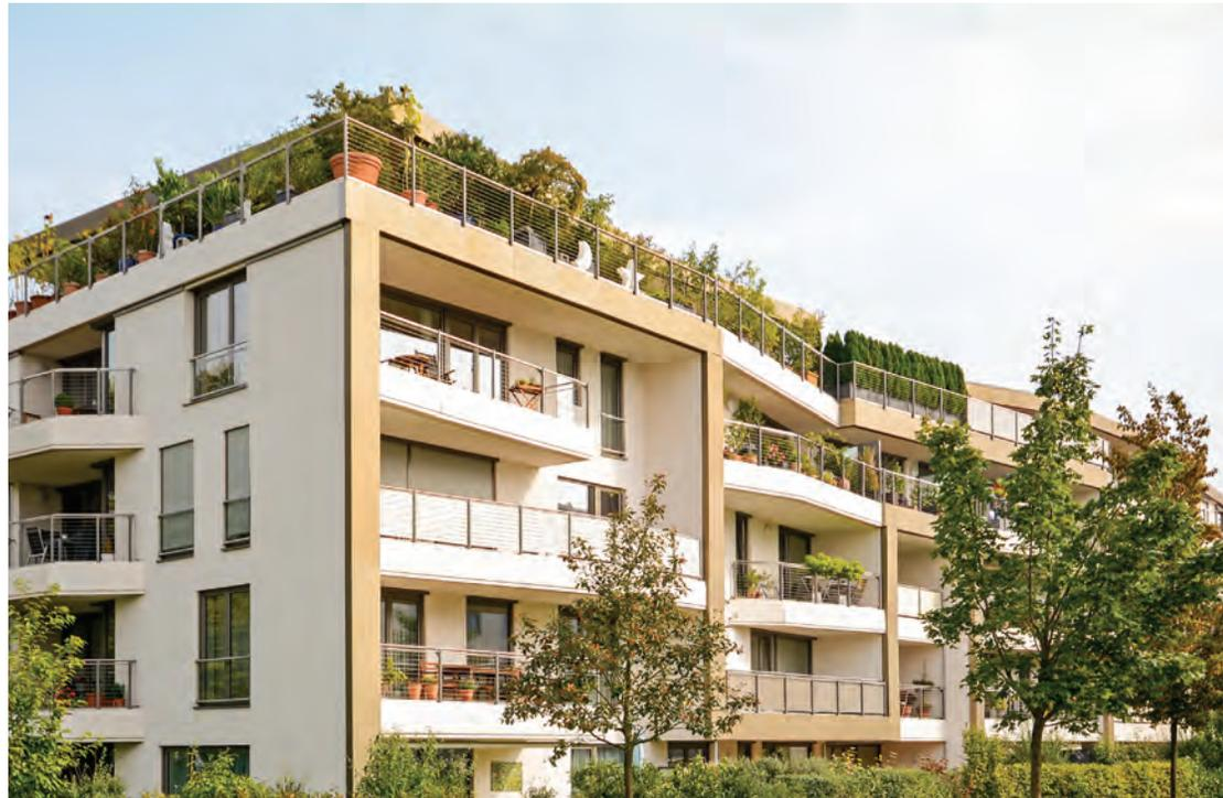
Green roofs are encouraged for additional amenity space and to reduce stormwater run off.
