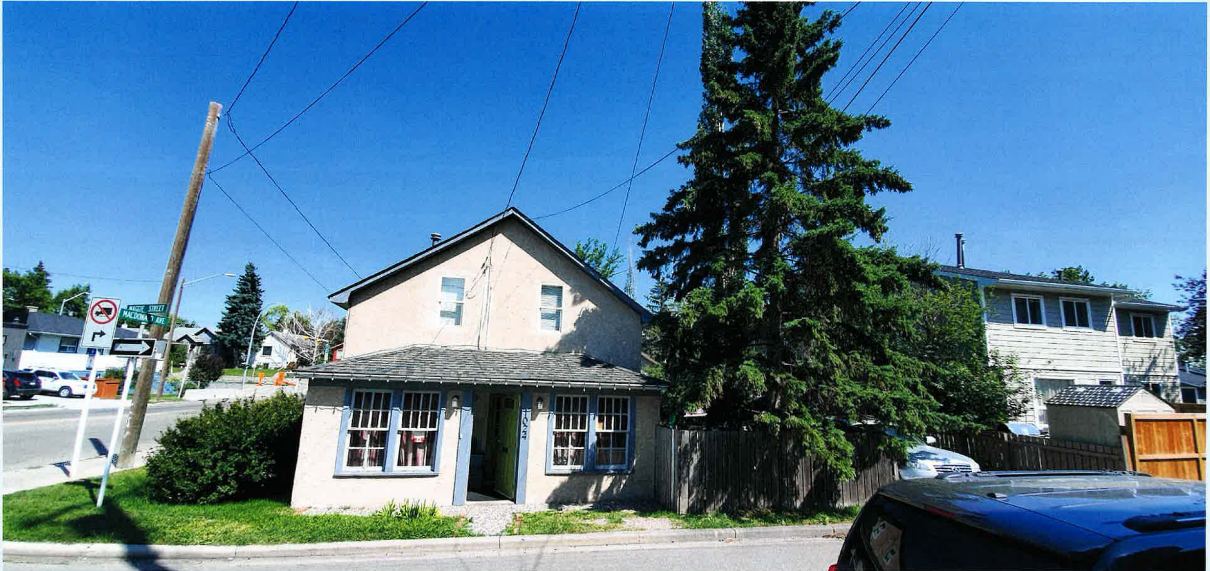
View of the subject site looking east
