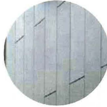
B1 - FIBRE CEMENT BOARD CLADDING
