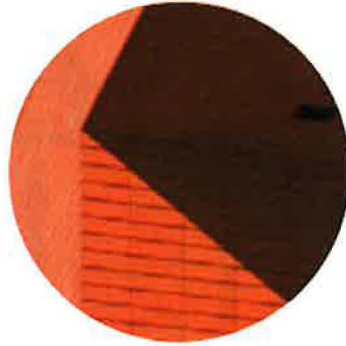
A2 - TERRACOTTA CLADDING & SOFFIT
