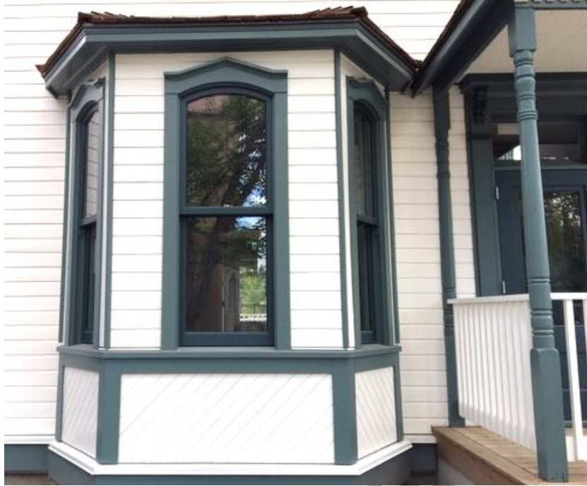
(Image 1.2: Hipped bay window with diagonal siding)
