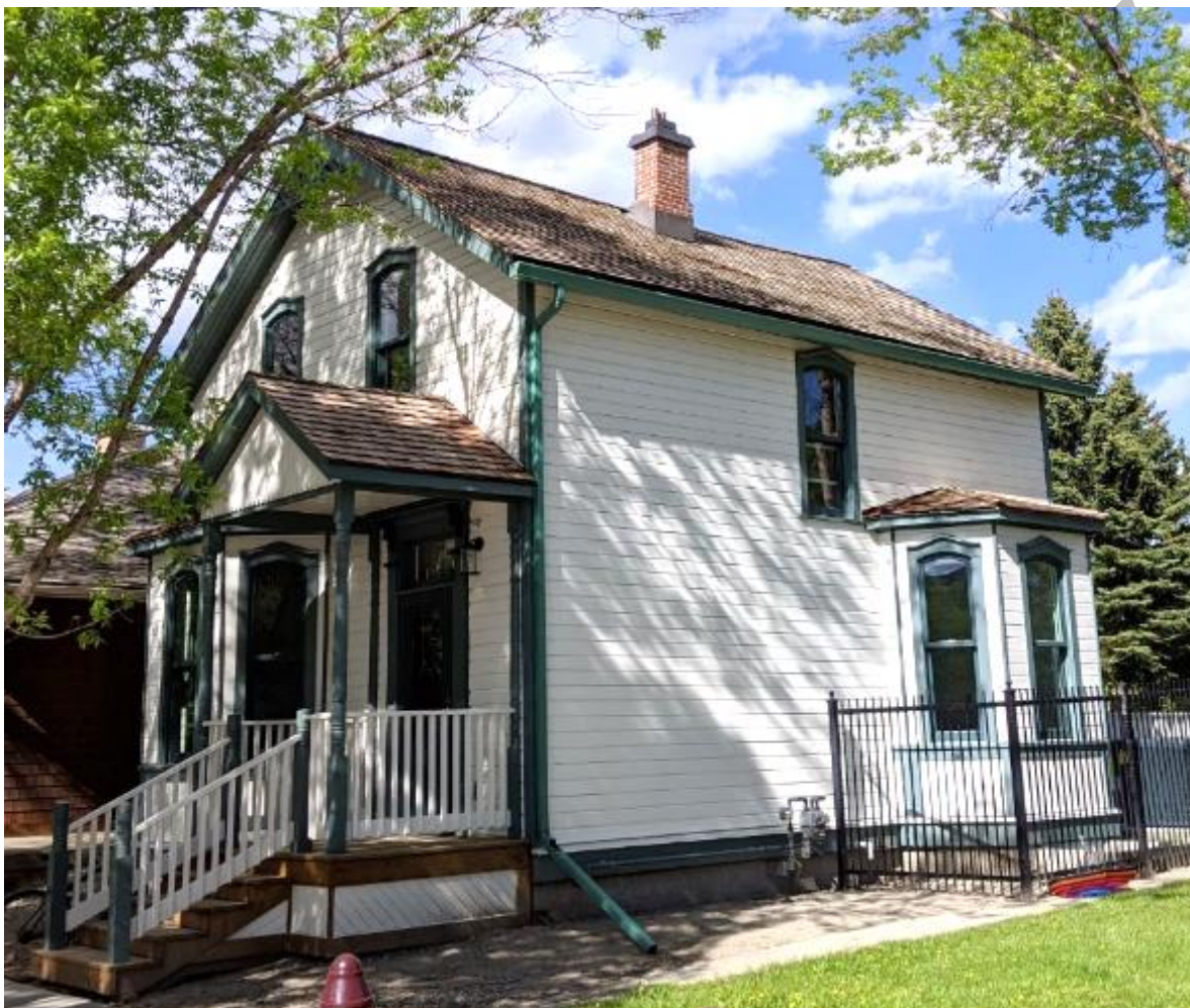
(Image 3.1: Oblique view of South façade)
