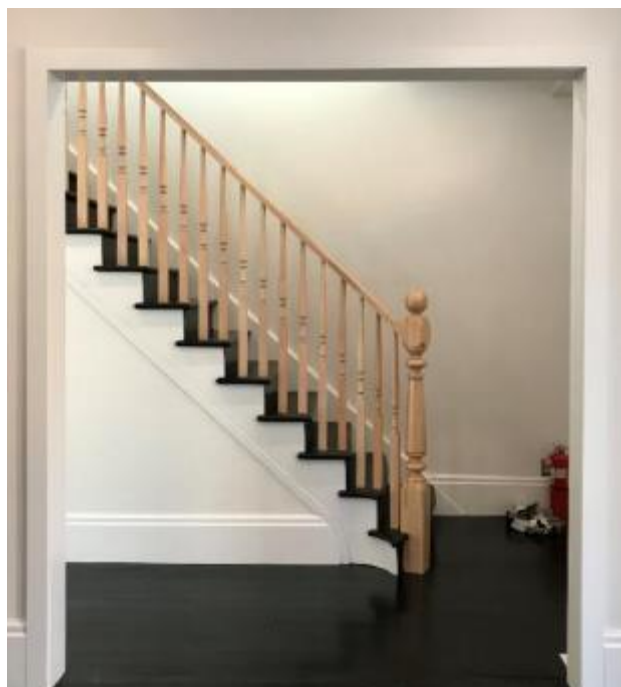
(Image 7.1: Balustrades and newel post)
