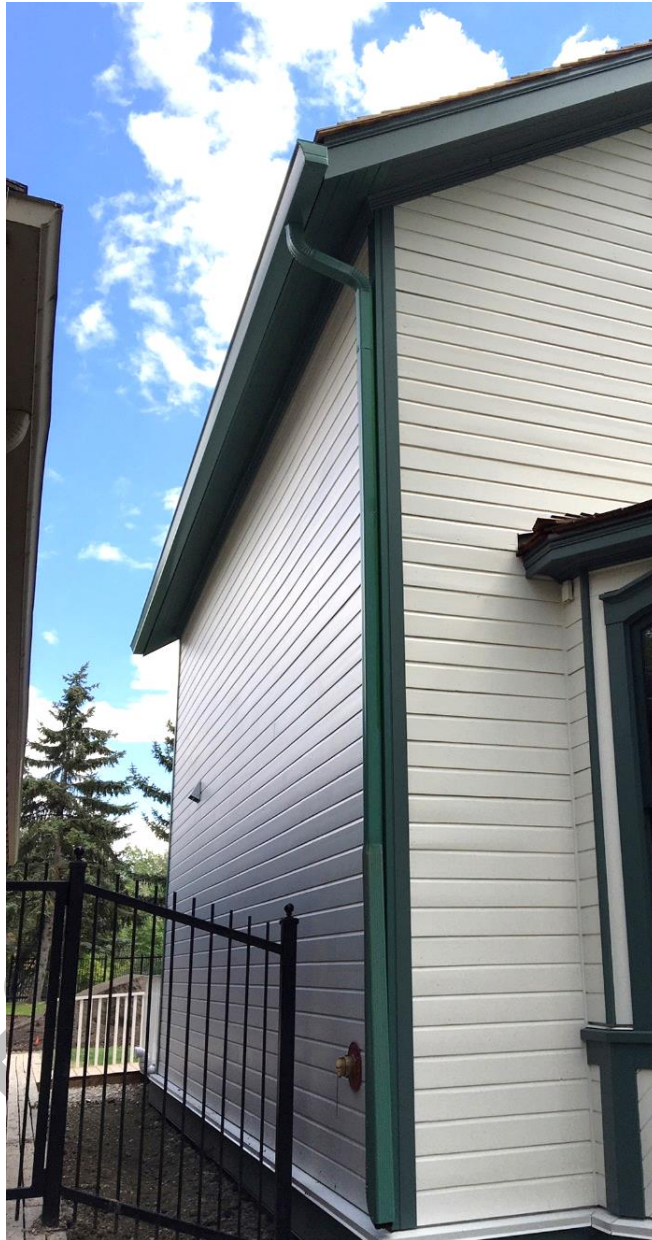
(Image 4.1: Oblique view of North façade)
