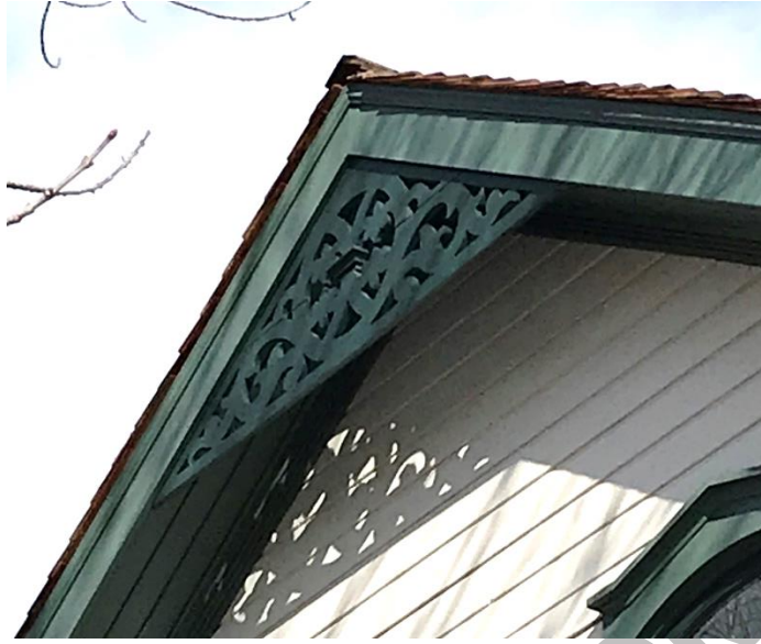
(Image 1.4: Fretwork detailing at roofline)
