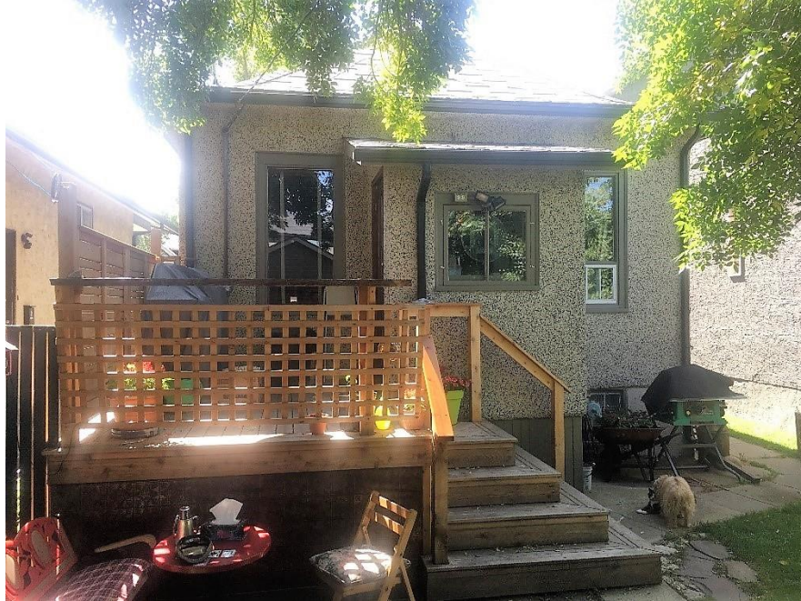
(Image 2.3: North façade including rear bay and fenestration)
