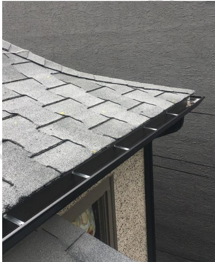
(Image 2.8: Detail of southeast corner of bell-cast (curved) roof)
