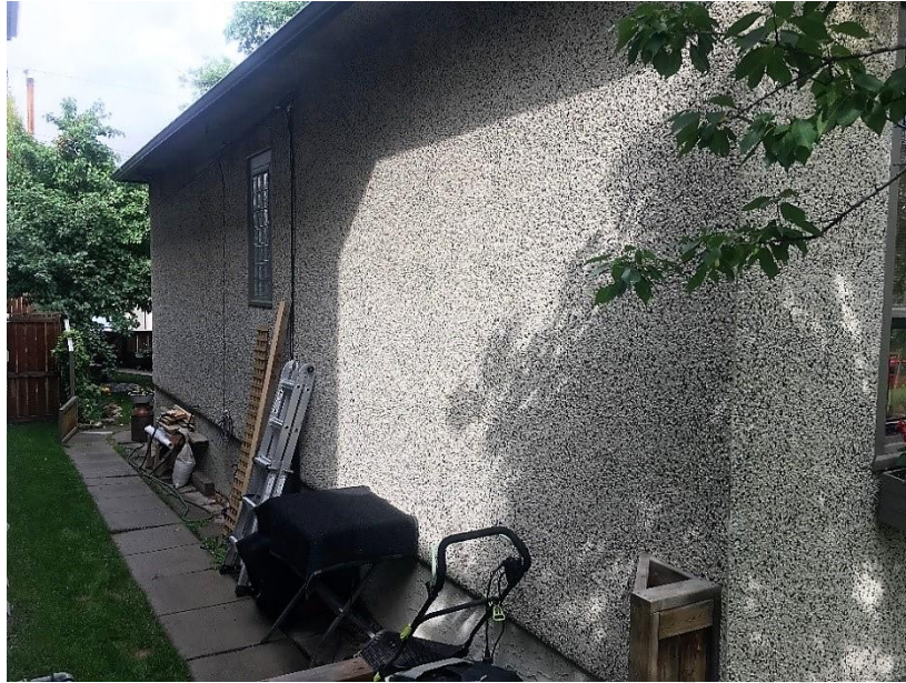
(Image 2.5: Oblique view of west façade including fenestration)
