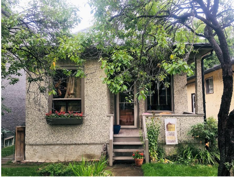
(Image 2.1: South façade)
