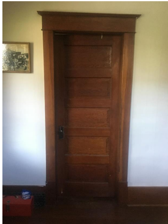
(Image 3.2: Example of typical 5 panel door and door casing in the hallway)
