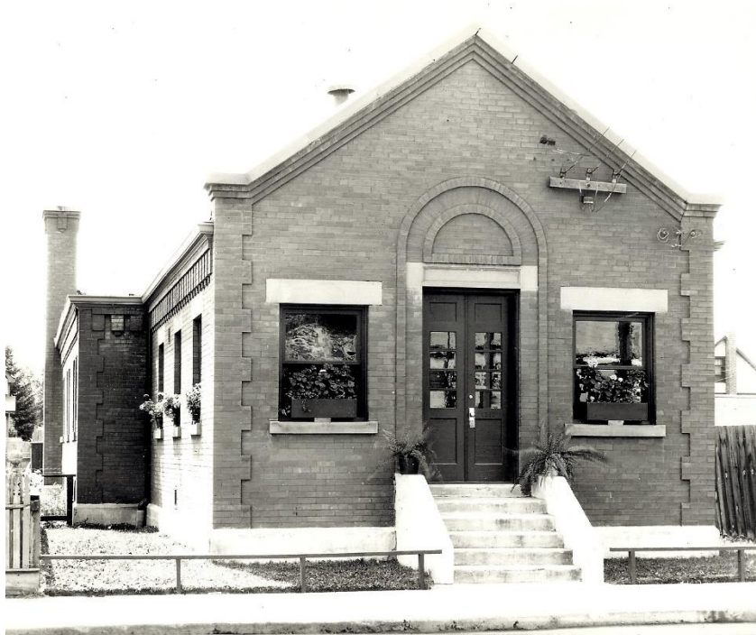
(Image 1.2: Historic image of north façade showing the original 1-over-1 sash windows and Roman arch above the central front entrance, ca. 1910-1920, Copyright AGT Archive)
