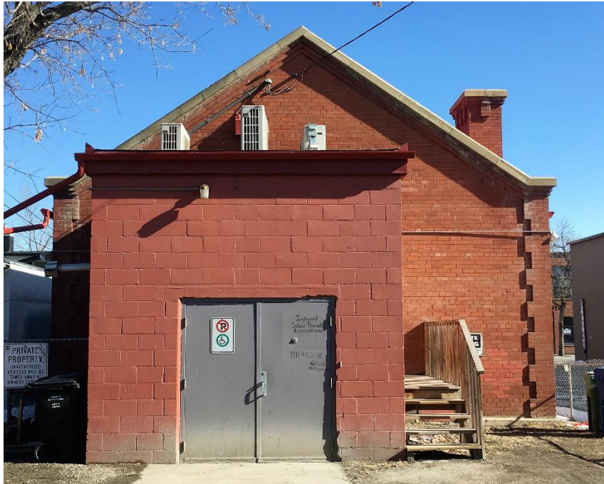
(Image 3.1: South façade with ca. 1955 cinder block rear extension)
