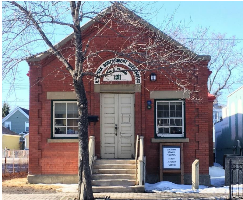
(Image 1.1: North façade)
