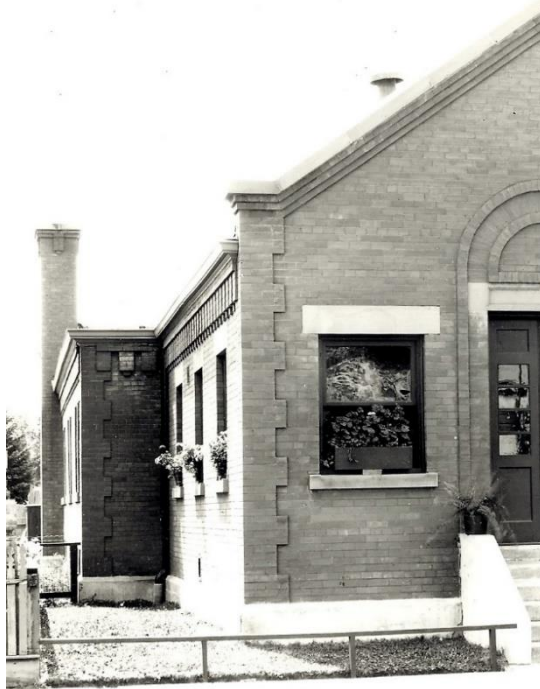
(Image 2.3: Historic image showing detail of quoins at building corner, 1910-1920, Copyright AGT Archive)
