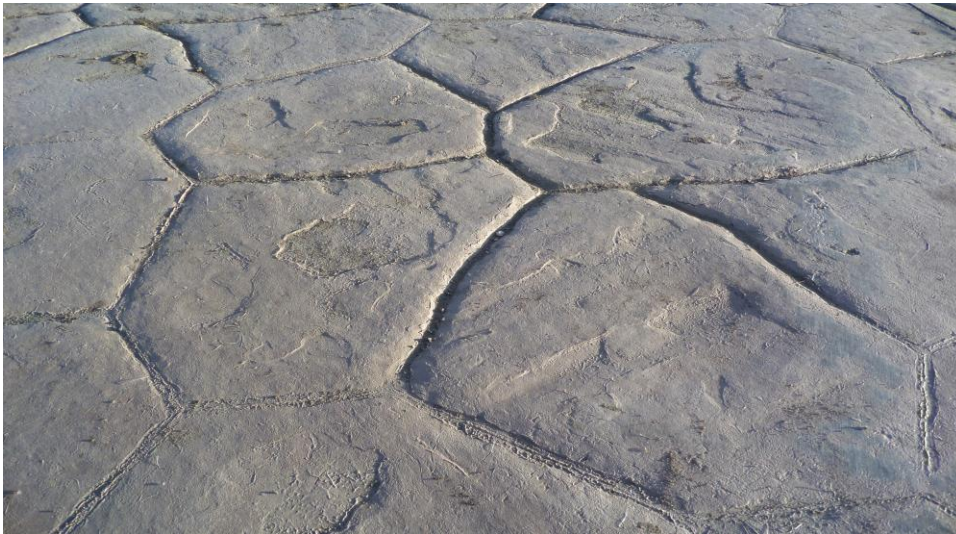
Figure 11: Decorative concrete in Auburn Bay, Calgary
