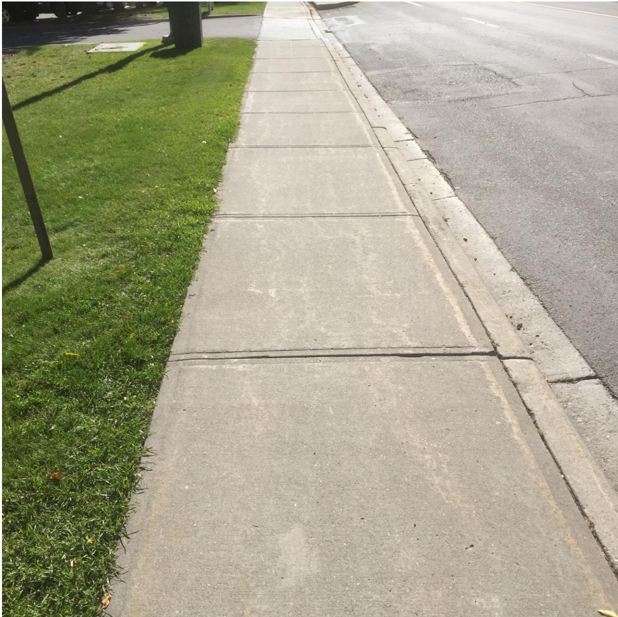
Figure 6: Example of Concrete Sidewalk in Very Good Condition
