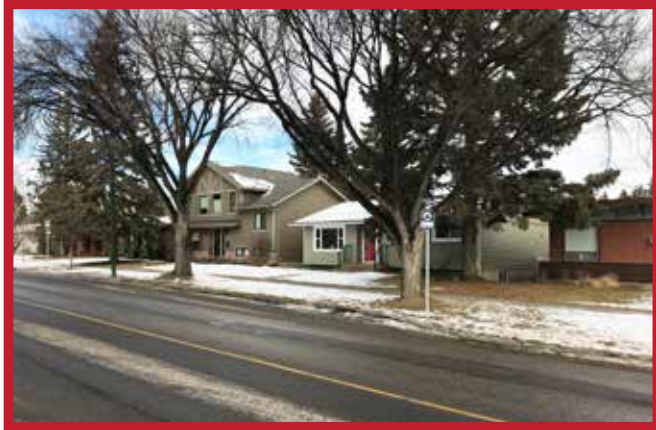
VARSITY RESIDENTIAL: FRONT PORCH CONDITION
