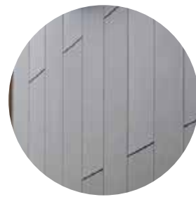
B1 - FIBRE CEMENT BOARD CLADDING
