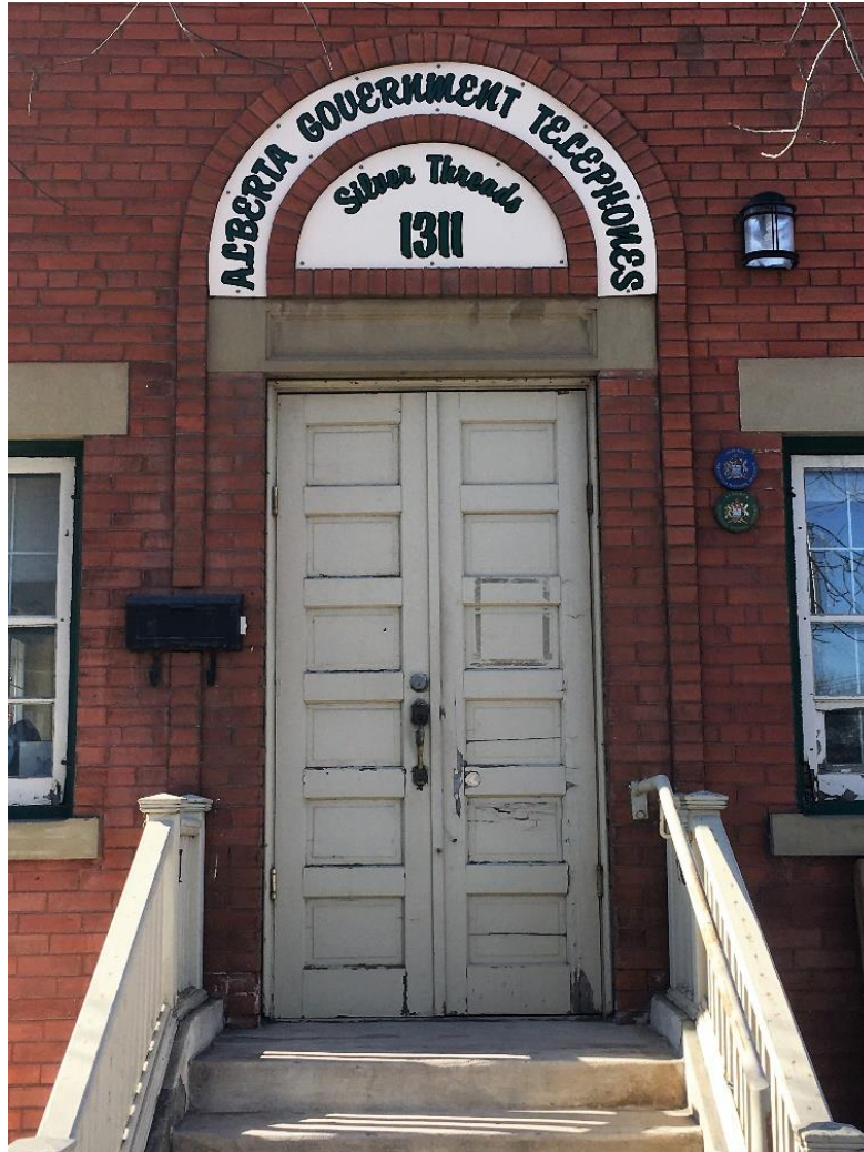
(Image 1.4: Detail of central front entrance with sandstone lintel and surmounted by brick relief in Roman-arch design)
