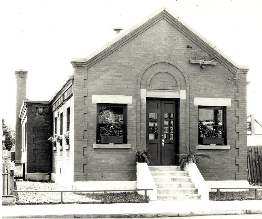
(Image 1.2: Historic image of north façade showing the original 1-over-1 sash windows and Roman arch above the central front entrance, ca. 1910-1920, Copyright AGT Archive)
