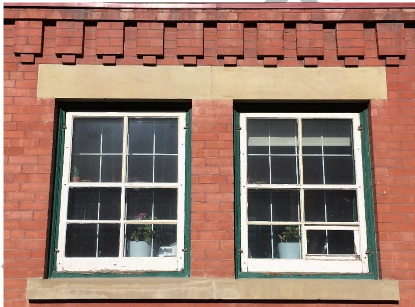
(Image 2.2: Typical fenestration and corbelled modillions on side elevations)
