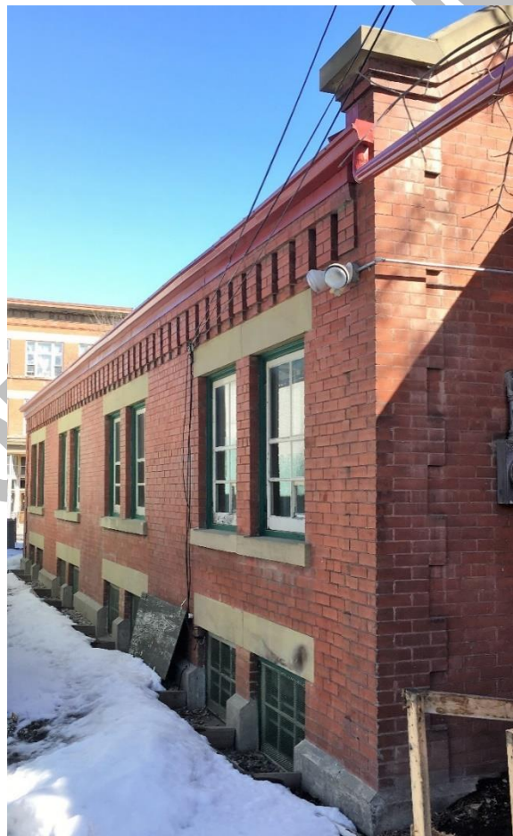
(Image 4.2: Oblique view west façade rear addition looking northeast)
