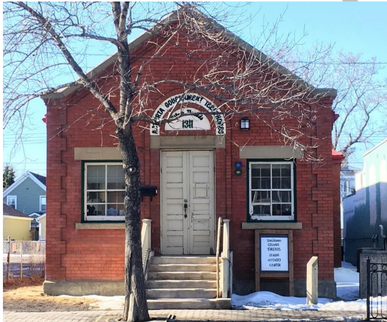
(Image 1.1: North façade)
