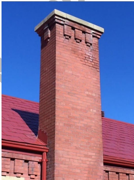
(Image 2.4: Detail of corbelled modillions and sandstone cap of red-brick chimney on east façade of rear addition)
