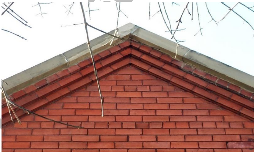
(Image 1.3: Detail of common bond pattern red brick with red-pigmented mortar and corbelled cornice at gable edge with sandstone cap)
