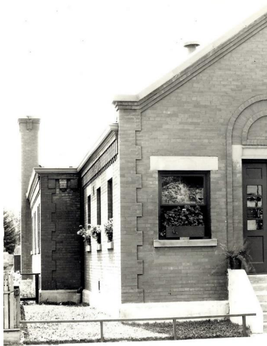
(Image 2.3: Historic image showing detail of quoins at building corner, 1910-1920, Copyright AGT Archive)
