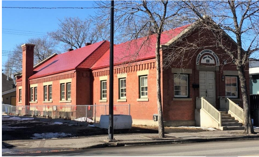
(Image 2.1: Oblique view of east façade with rear addition added 1912-1913)
