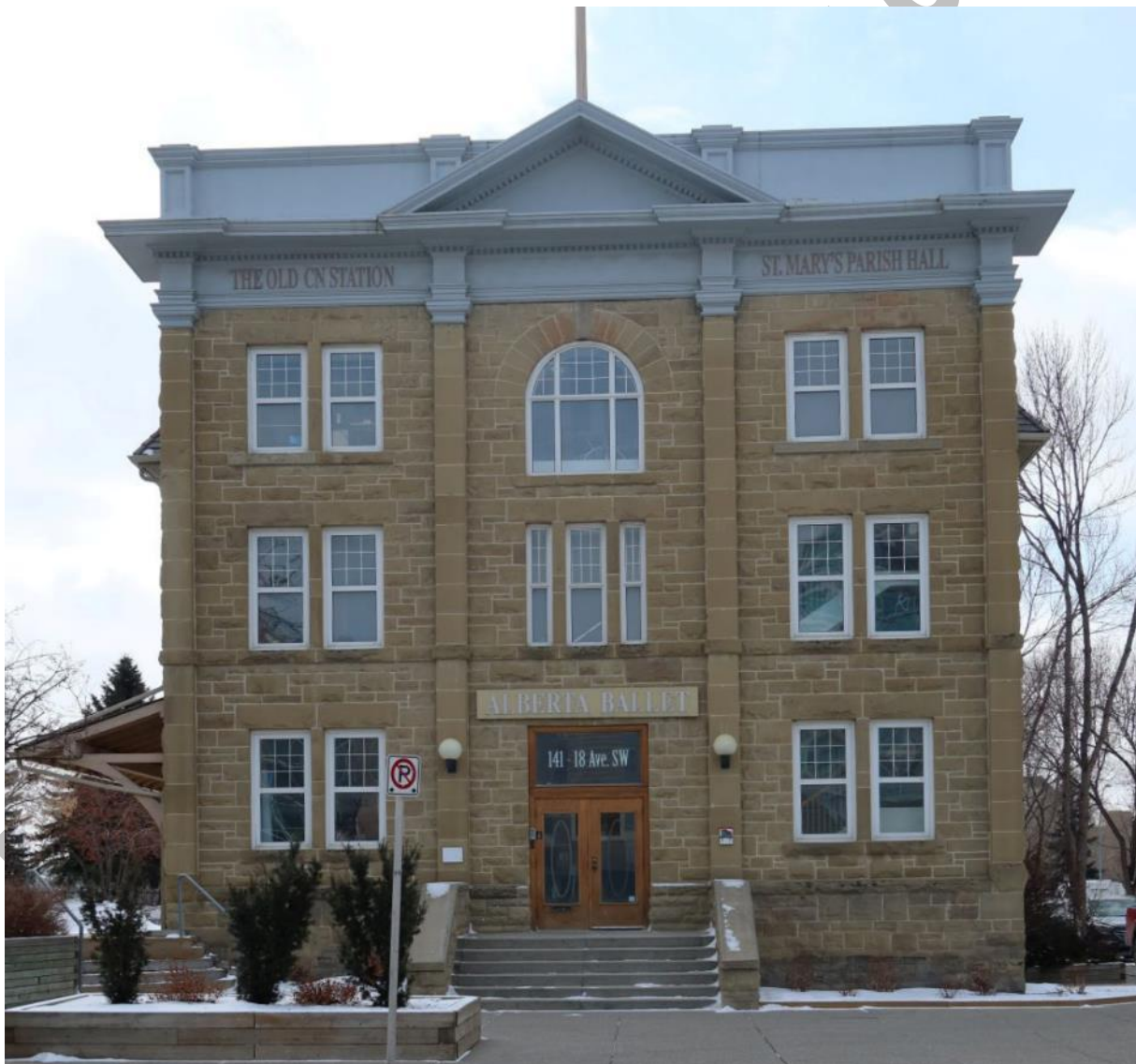
(Image 1.1: North façade)
