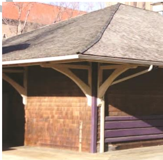
(Image 5.2: 1951 Wood Frame Freight Shed)
