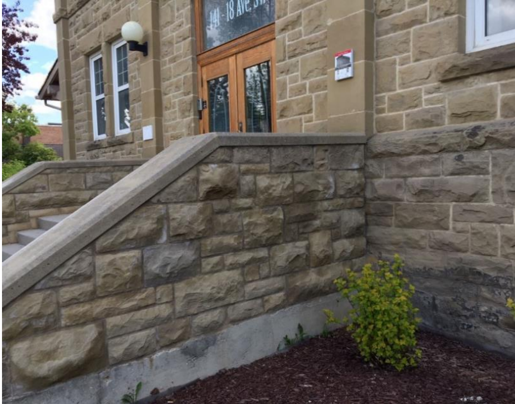
(Image 1.2: Rubble-coursed sandstone foundation and sandstone wall)
