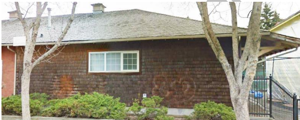
(Image 5.4: 1951 Wood Frame Freight Shed west façade)
