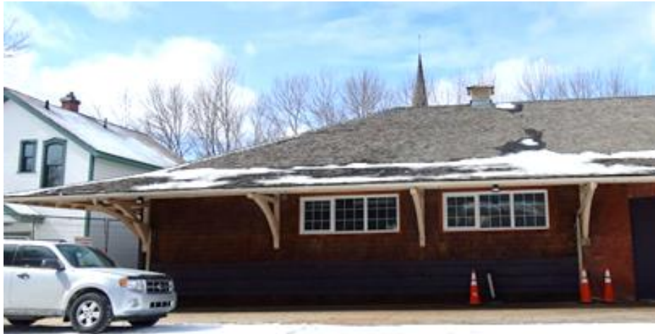
(Image 5.3: 1951 Wood Frame Freight Shed east façade)
