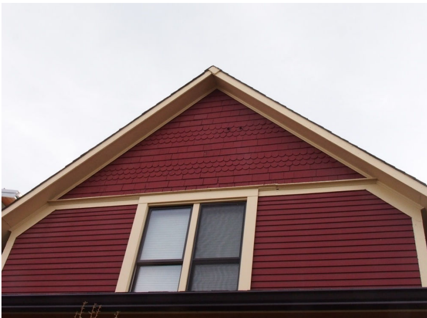
(Image #2.6 – Front gable of the west façade with fish scale detailing)
