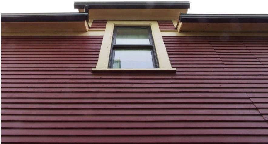
(Image #2.7 – Low-pitch shed-roof dormer on north façade)
