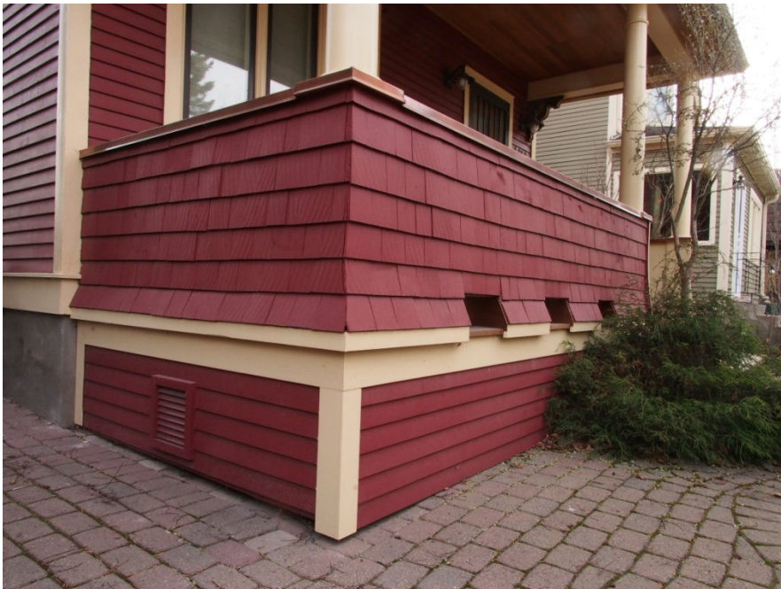
(Image #2.10 – Solid balustrade and shingle cladding of front porch)
