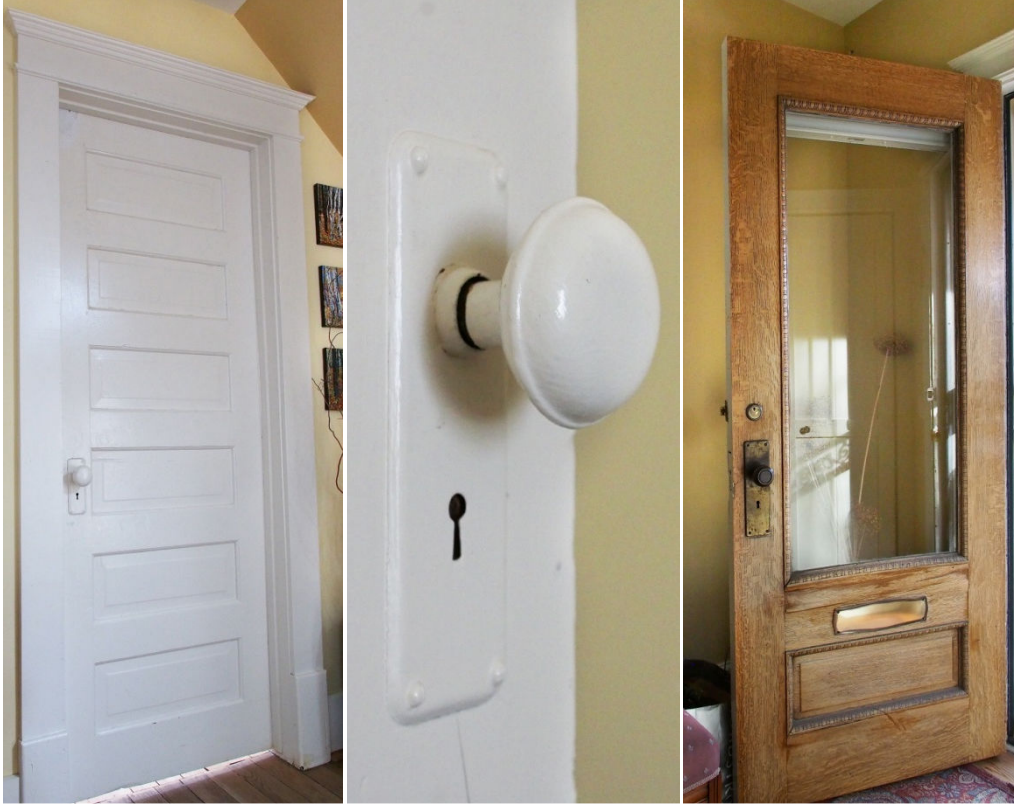
(Image #3.4 – Left: Example of original interior doors (one of five shown); Centre: Detail of interior door hardware; Right: Original front door and hardware)
