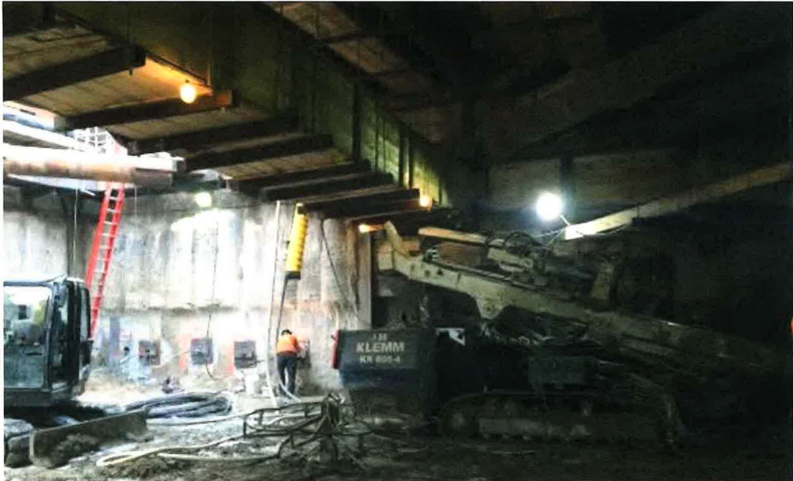
Example of large utilities suspended in excavation
