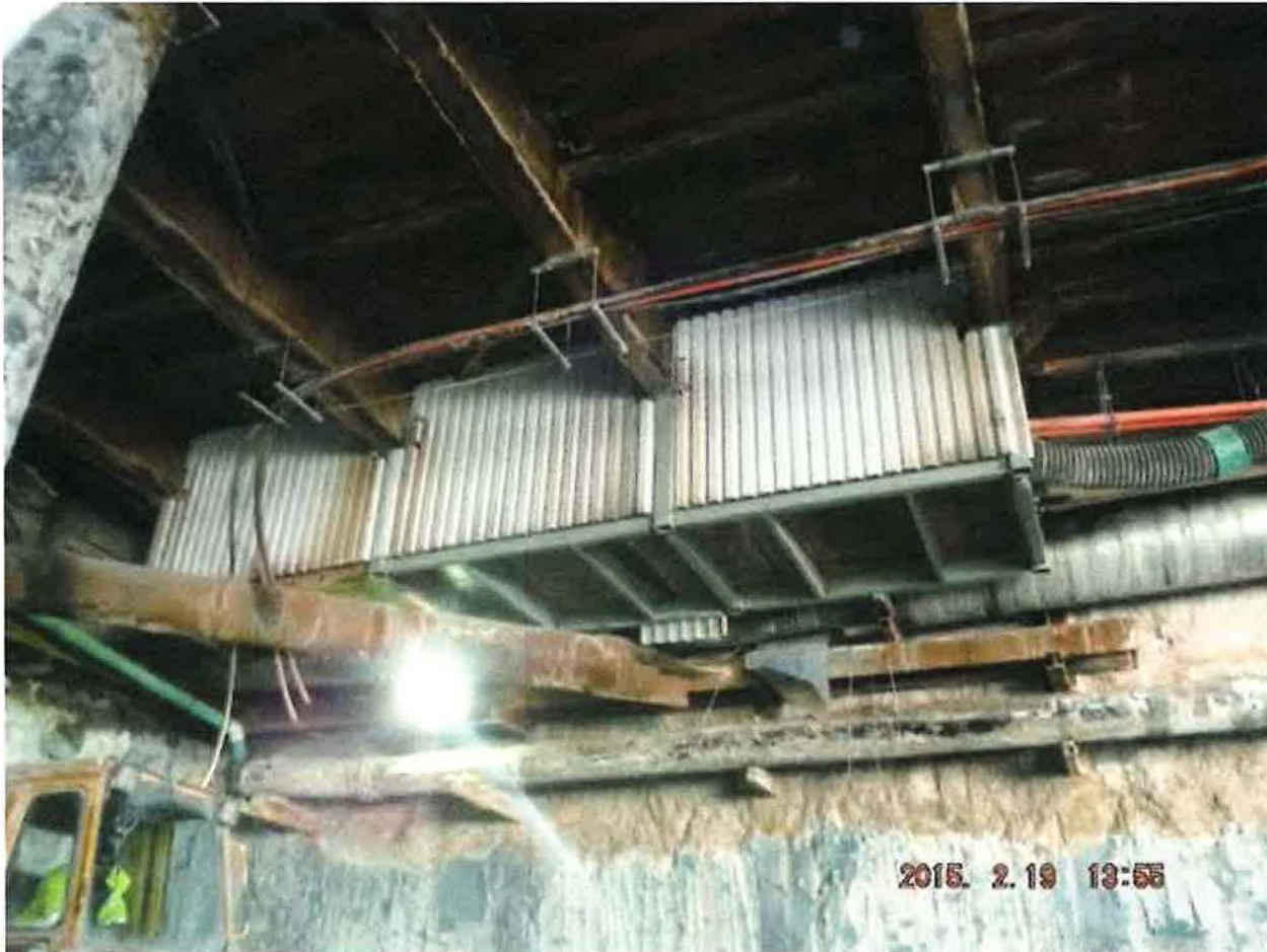
Example of large utilities suspended in excavation
