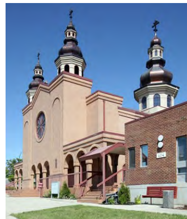
St. Vladimir's Ukrainian Orthodox Church and Cultural Centre (1977) Identified heritage resource— currently without legal protection preventing significant alteration or demolition
