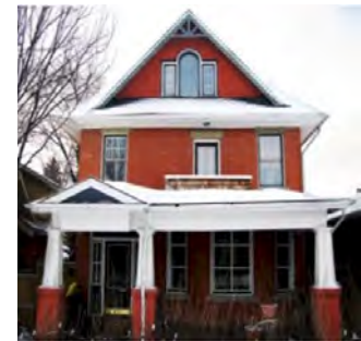
Robert and Mary Taylor Residence (1912) Municipally-designated heritage site
