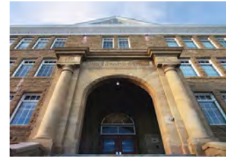
King Edward School (1912) Example of a heritage site listed on the Inventory of Evaluated Historic Resources
