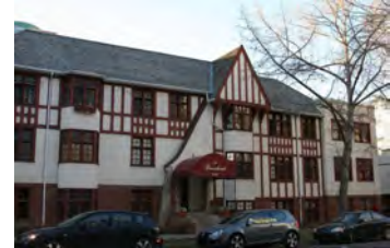
Barnhart Apartments (1929) Transferred density within Calgary's Beltline community
