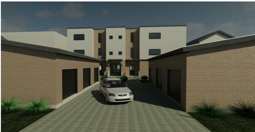
Exterior (South face)
