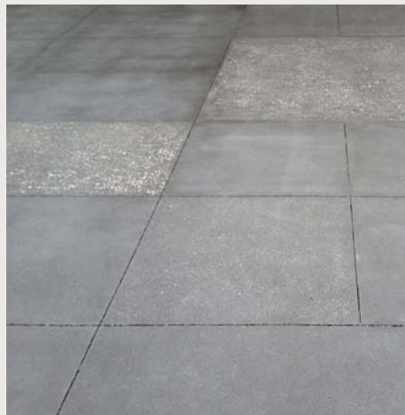
Cast-in-place Pigmented sawcut Concrete
