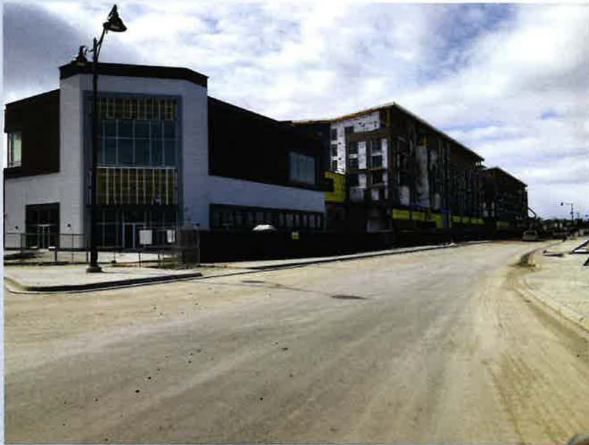
West view of Block I along Na'a Drive SW
