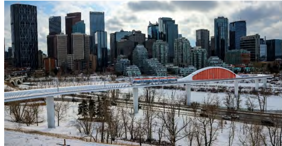
Tied arch bridge rendering. A tied arch bridge utilizes a moderate vertical upstand spine in the centre of the bridge to provide vertical support for a main span over the Bow River. A constant depth viaduct would be used on either side of the main span crossing Prince's Island Park and Sunnyside Bank Park.
