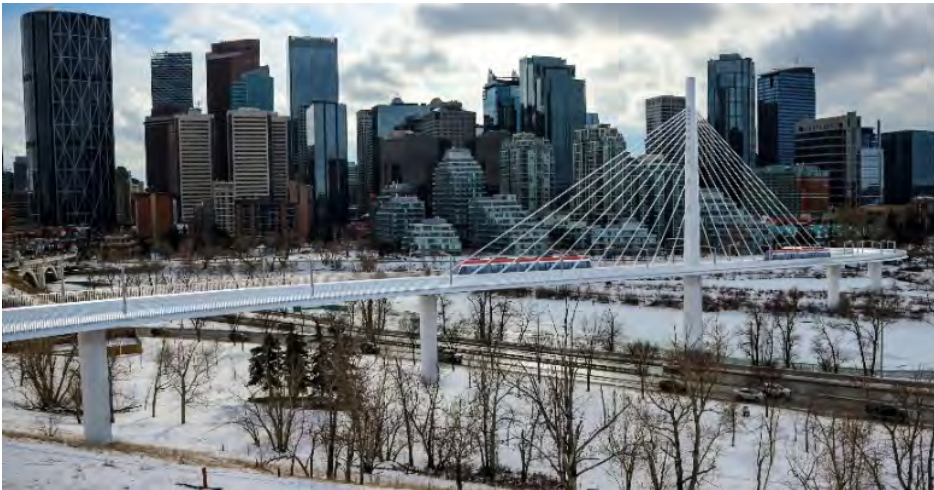
Cable stayed bridge rendering. A cable stayed bridge utilizes a large singular vertical pylon in the centre of the Bow River to support two cable stayed spans on either side. On the north side, the span extends over the Memorial Drive, and on the south side, it extends over Prince's Island Park. This type of structure has a larger visual impact.
