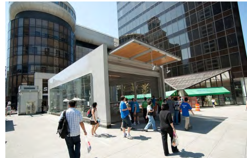
Example of what a stand-alone station entrance might look like, showing Canada Line in Vancouver.
