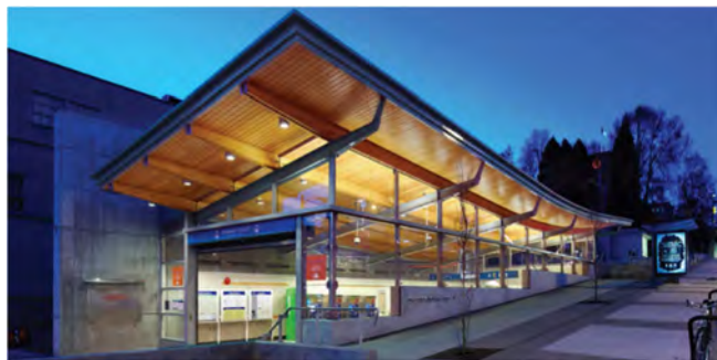
Example of what an underground station entrance might look like before its integrated into a development, showing Broadway Station in Vancouver.
