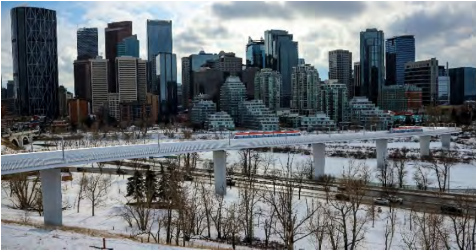
Constant depth viaduct rendering. A constant depth viaduct is a simple bridge structure with evenly spaced piers and a constant depth structure between the piers. This type of structure allows for smaller piers, but as a result, requires that the piers touch down more frequently than other bridge types.
