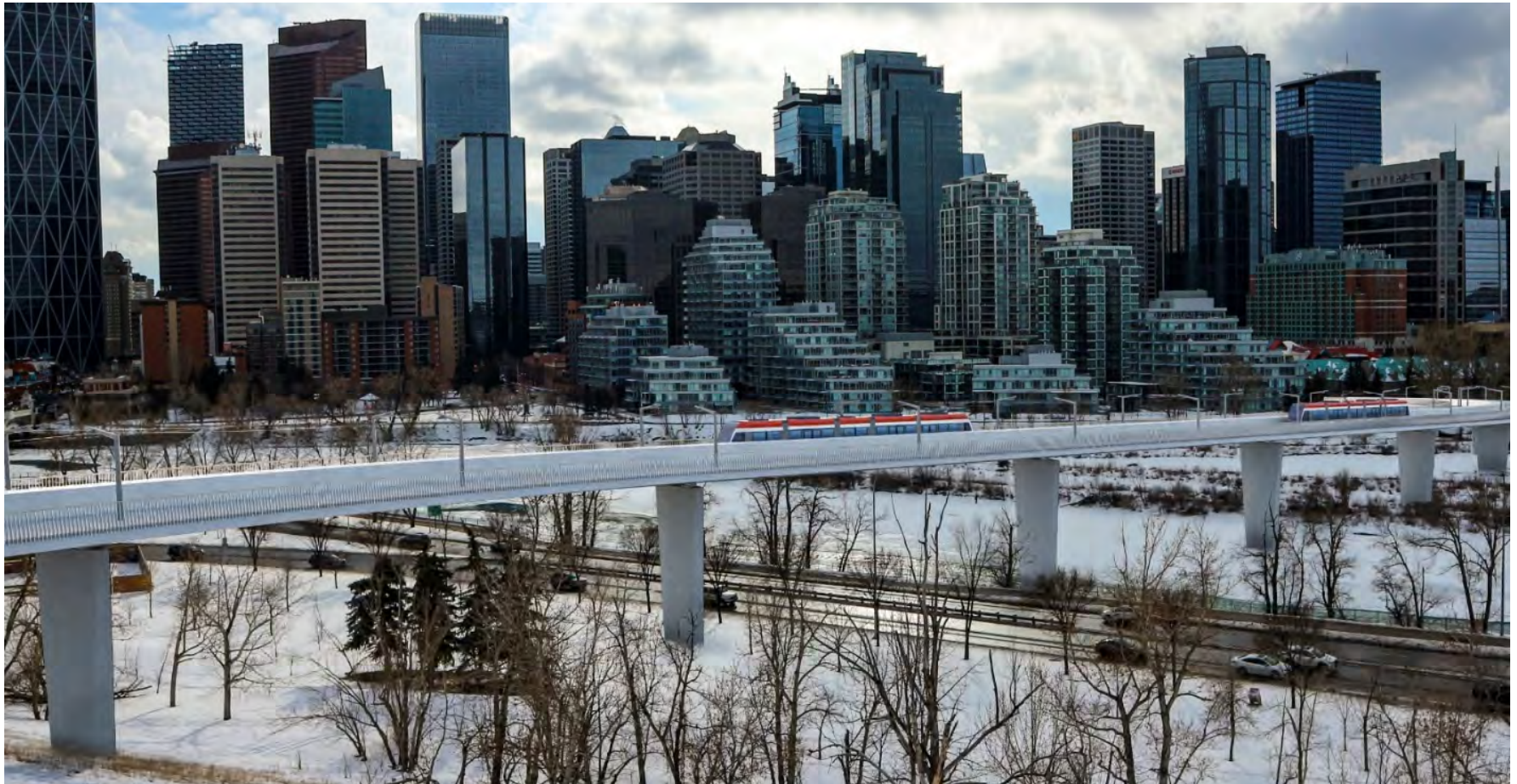
Rendering of LRT bridge (constant viaduct structure), as viewed from McHugh Bluffs on north side of Bow River.
