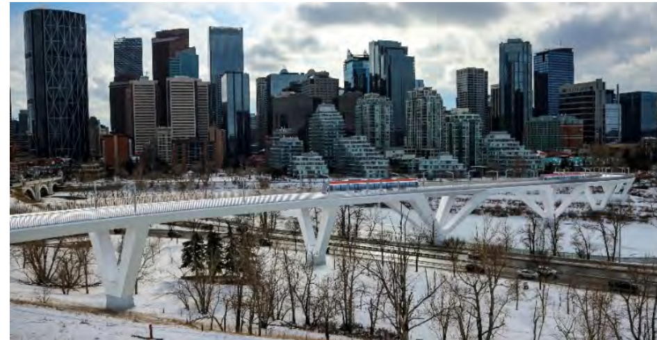
Trestle bridge rendering. A trestle pier viaduct is a simple bridge structure with evenly spaced v-shaped piers. The v-shaped piers reduce the clear span between piers which allows for a shallower bridge deck. The unique shape of the piers would require additional constructability considerations.
