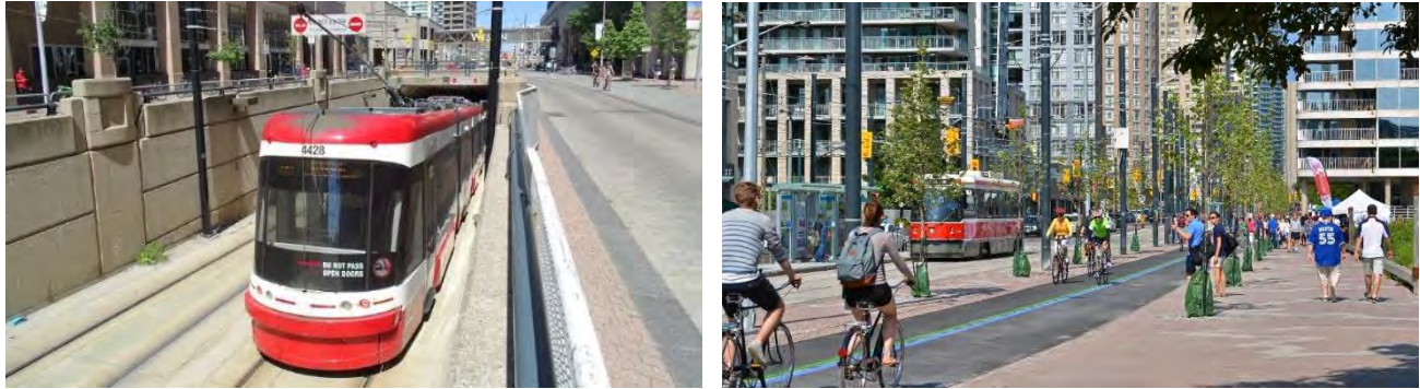
Figure 77: (Left) Streetcar Portal along Queens Quay in Toronto; (Right) The multi-modal streetscape and public realm design along Queens Quay
