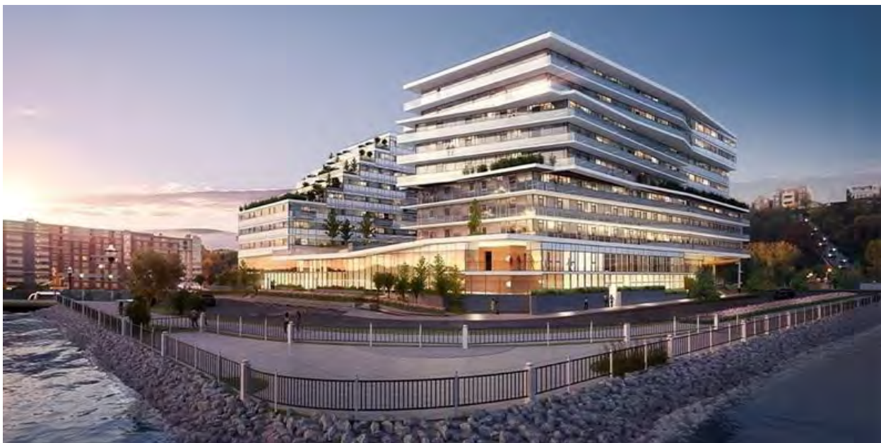
Figure 347 – Development at Port Imperial (Source: Avora at Port Imperial)
