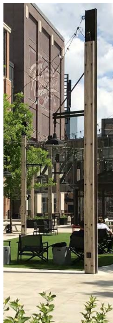
PEDESTRIAN LIGHTS LOCATION: PROMENADE MARKET STREET
