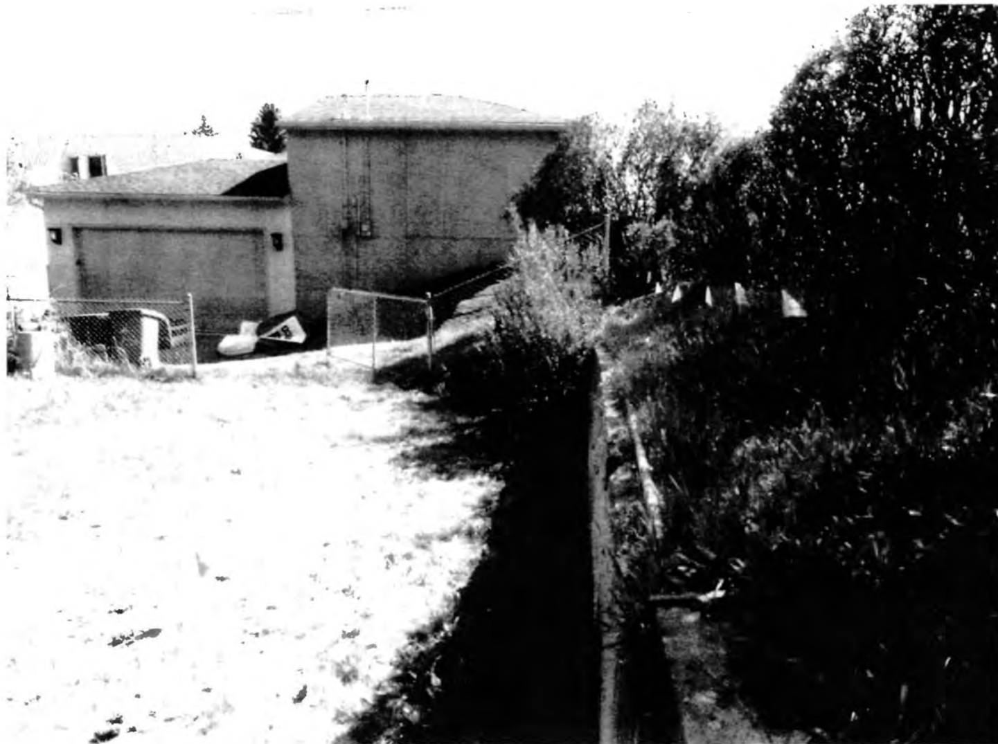
View from subject lot facing rear laneway. Note the existing retaining wall and grade differential from west property line (green flags).
