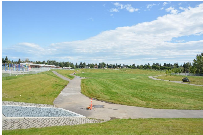
THE BRAESIDE DRY POND WILL ADDRESS FLOODING CAUSED BY RAINFALL IN THE COMMUNITY OF BRAESIDE WHILE ALSO SERVING AS COMMUNITY RECREATION FACILITIES WHEN NOT STORING STORMWATER
