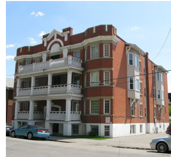
Colgrove Apartments (1912) Identified heritage resource— currently without legal protection preventing significant alteration or demolition
