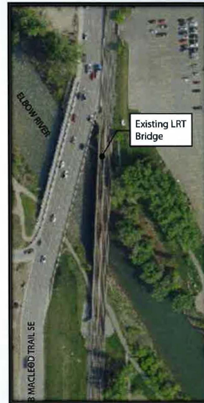
EXISTING LRT BRIDGE
