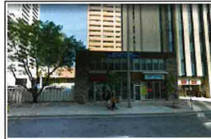
VIEW OF SITE FROM FRONT N78
