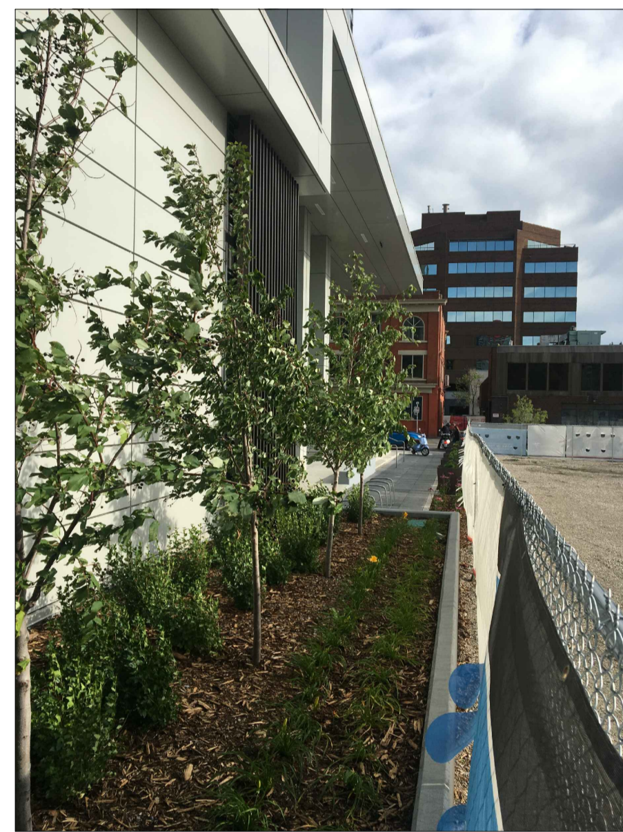
northeast corner of site looking south - showing adjacent condition
