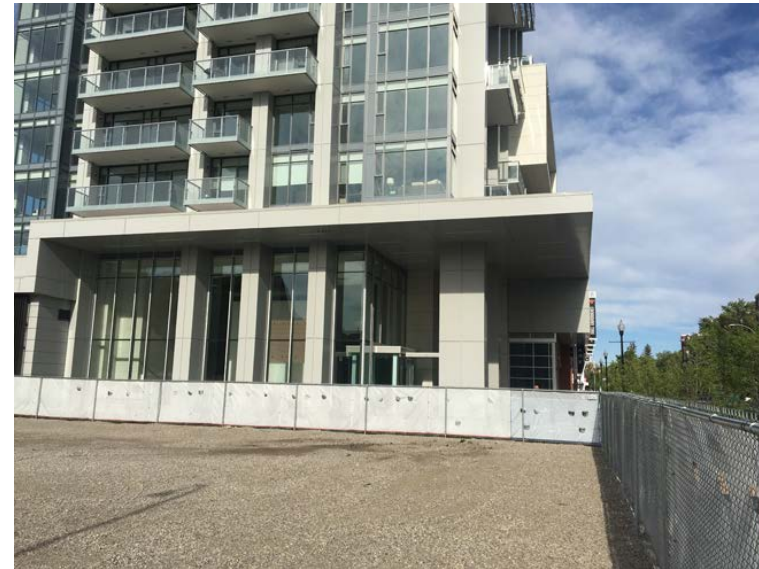
fig. 8 - site is directly adjacent the western edge of the BOSA Royal condominium building
