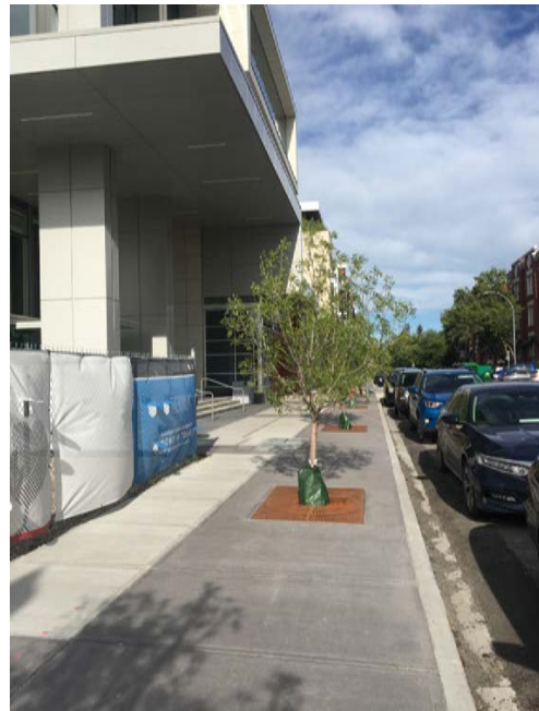
fig. 11 - sidewalk condition along 16th ave. sw
