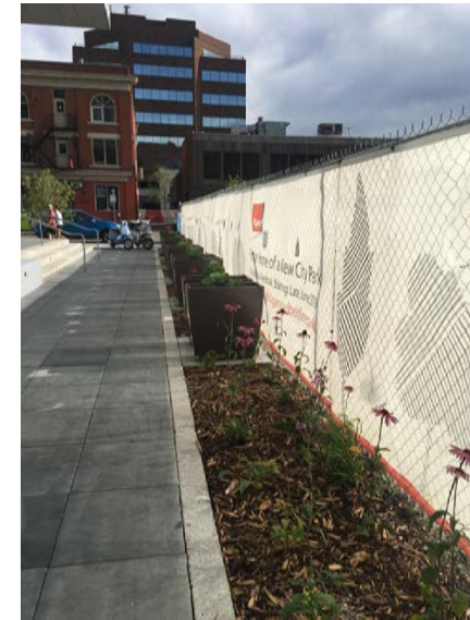
fig. 9 - interface with adjacent condo building
