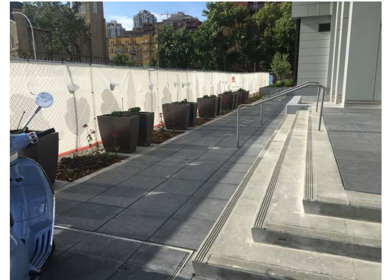
fig. 10 - interface with adjacent condo building
