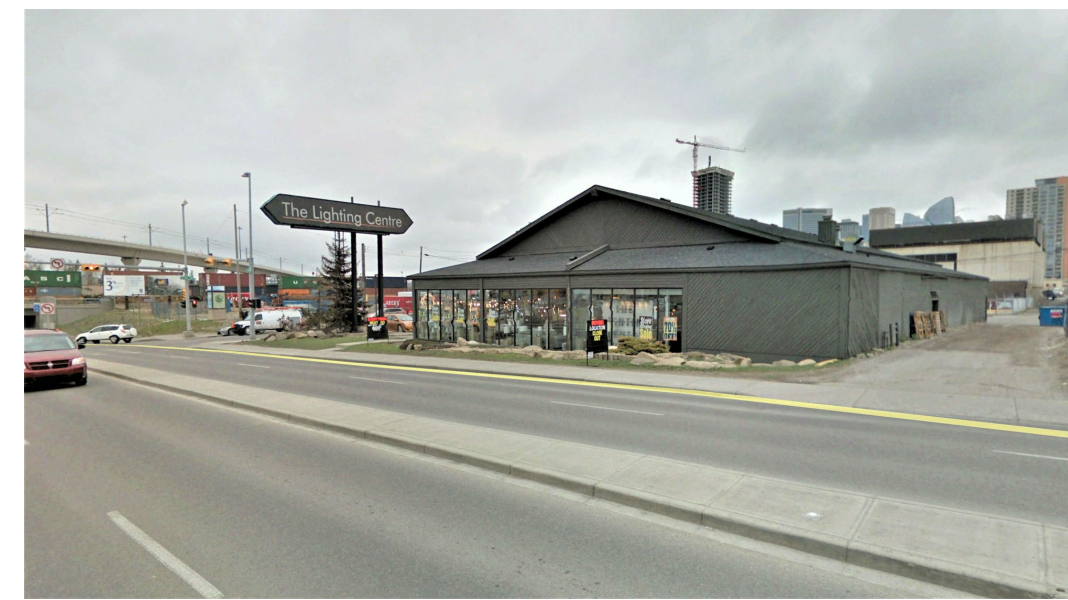
1. VIEW FROM SW LOOKING NE
