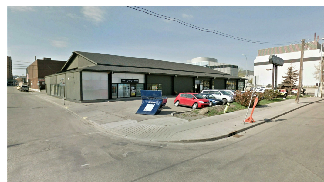
3. VIEW FROM NE LOOKING SW
