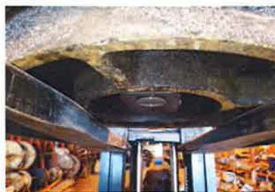
Transit Manhole Monitoring
