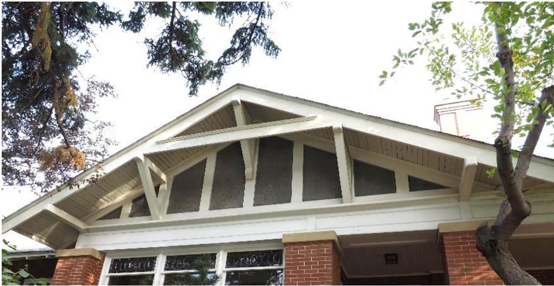
(Image 5.1: Detail of the north gable end; example of the tongue and groove soffits)
