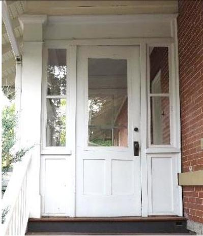
Image 4.3: Porch entrance trimmed with wooden paneling; wood door flanked by side-lites
