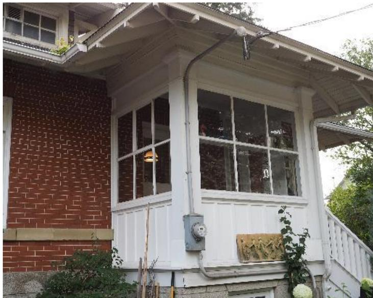
(Image 4.2: Enclosed porch trimmed with wooden paneling; wooden balustrade; six-lite windows)
