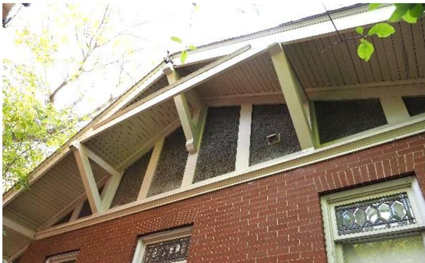
(Image 5.2: Detail of the north gable end; example of the tongue and groove soffits)
