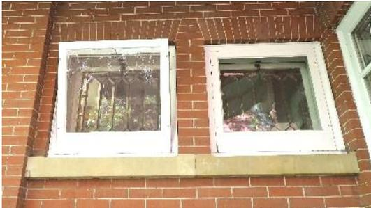
Image 2.3: Detail showing two of the three matching hopper windows with decorative beveled glass
