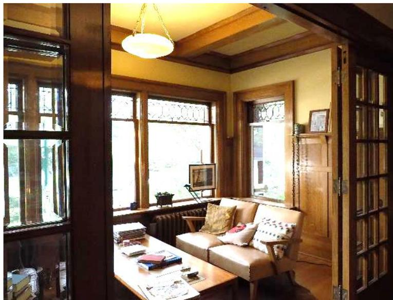
(Image 7.1: View into sun room with wood paneling, wood beams; wood room partition and French doors, both with beveled glass)
