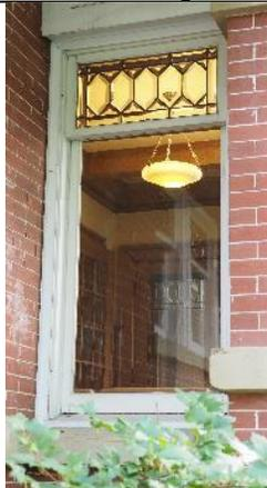
Image 3.5: Hung unit with decorative beveled glass transom, positioned on the east side of the gabled extension
