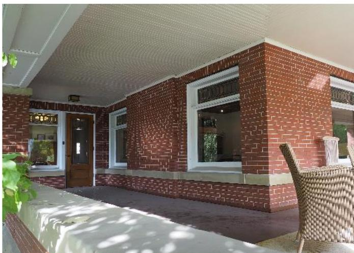
(Image 3.2: View looking northwest at the open wrap around porch with with wooden tongue-and-groove ceiling; continuous sandstone band; side entrance)
